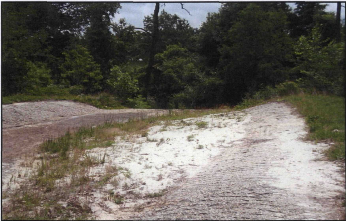
View east: Stormwater flume to Elevenmile Creek
