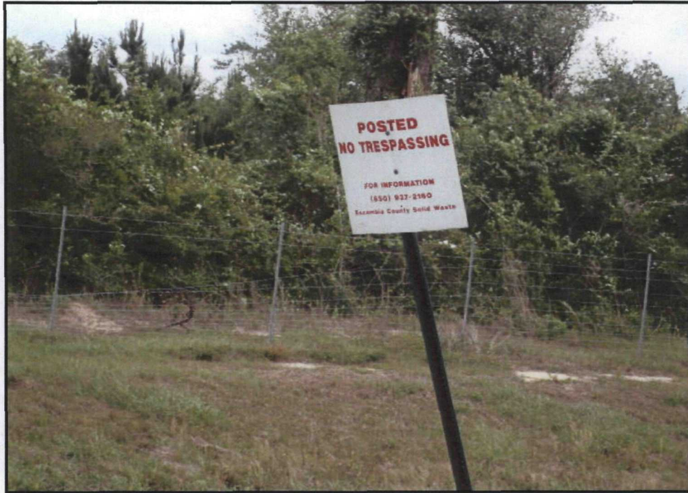
View north: Sign located on northern portion of landfill and damage to fence.
