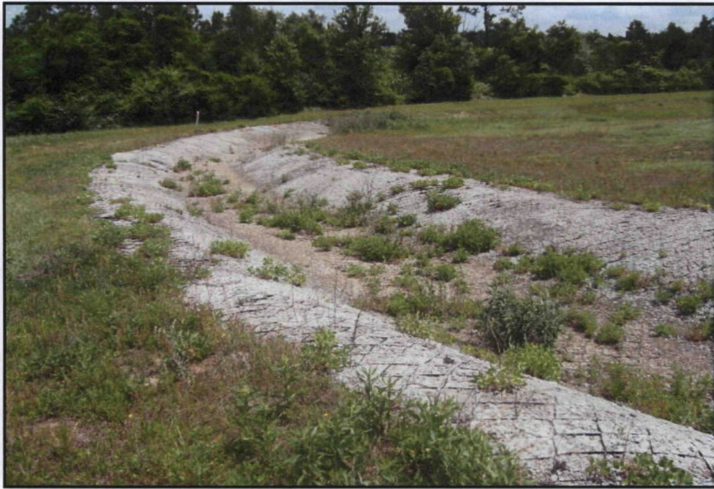
View northeast: Typical stormwater flume located on southern portion of landfill.
