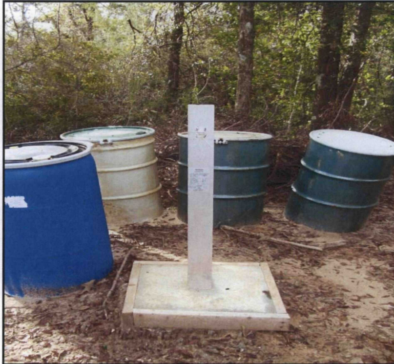
Newly constructed monitor well
