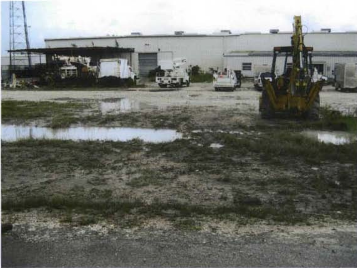
Equipment staging area east of the Miami Drum Services Site
