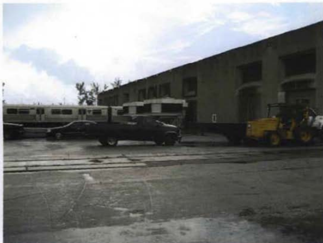
Train maintenance garage at rail yard
