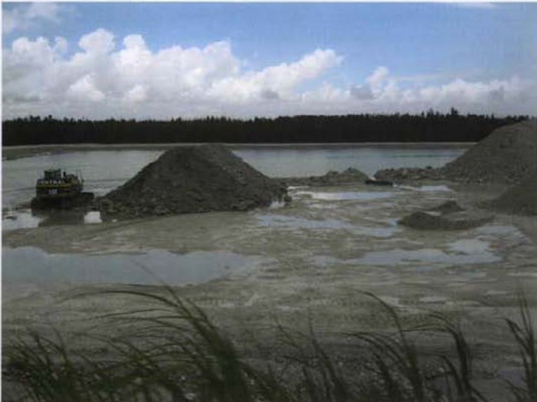
Settling ponds for WTP solids, located near the Northwest Wellfield
