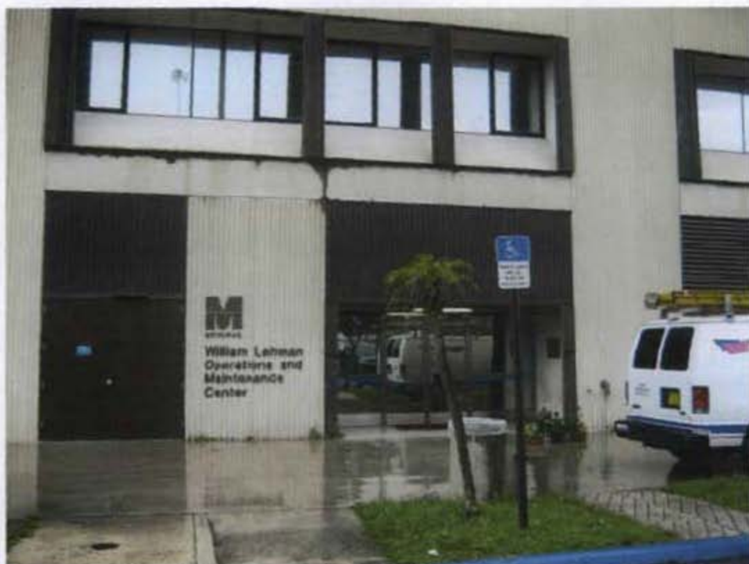
Entrance to rail maintenance yard office building
