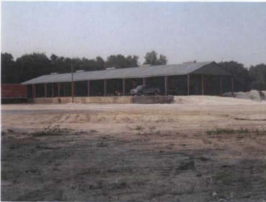
Former production building at the TCC Site being prepared for reuse as a commercial storage facility.
