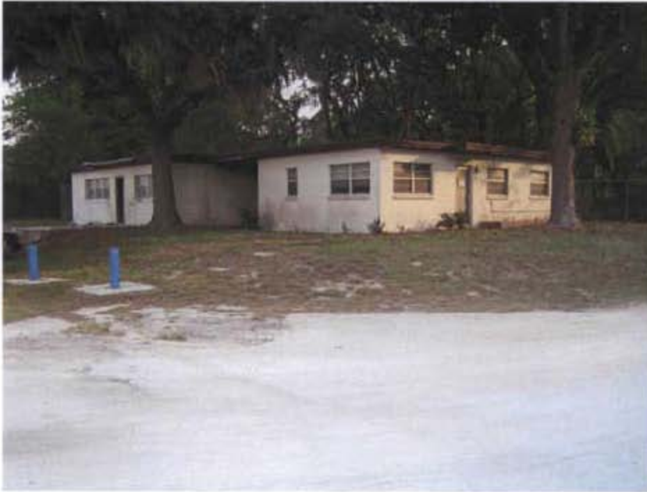
Former TCC office building. MWS-13 & MWF-13 on left.
