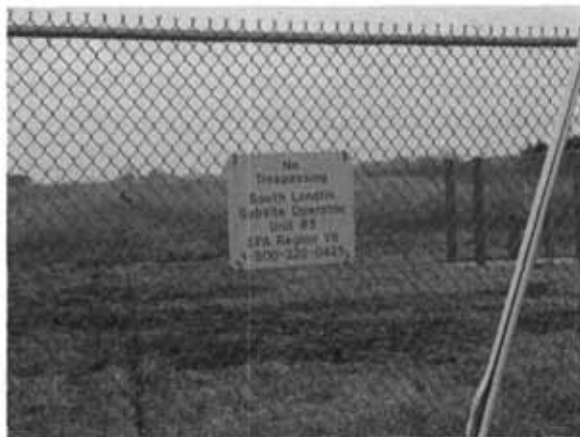
Figure 14 – South Landfill Subsite – completed landfill cap and fence surrounding subsite.
