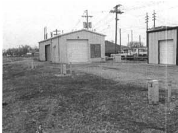
Figure 11 – Second Street Subsite – Ground water treatment and SVE system.
