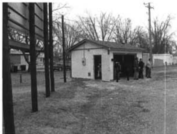
Figure 10 – Colorado Avenue Subsite – Phase III, East Highway 6 IWA system.
