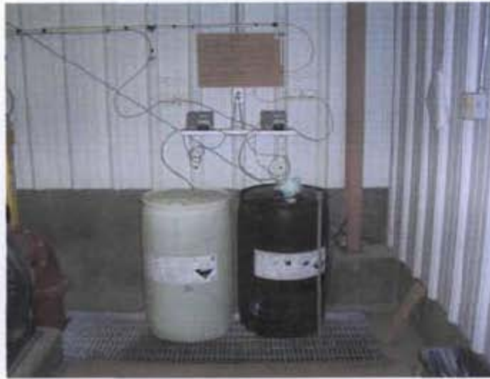
Photo 5: Chemical Treatment for the Drinking Water
