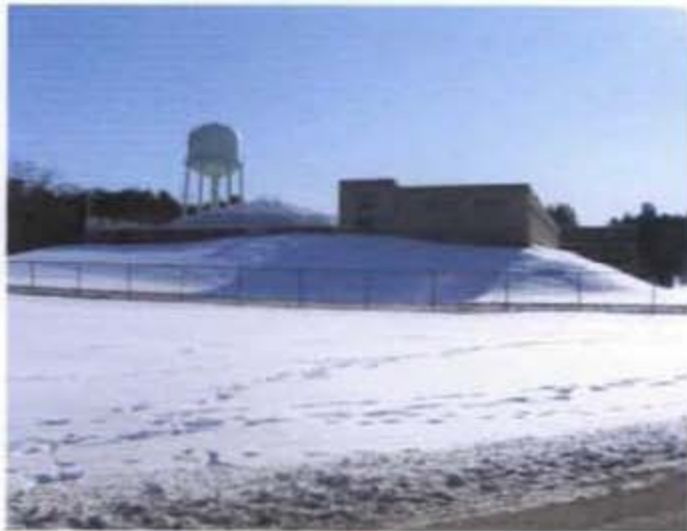
Photo 10: Water Treatment Plant
