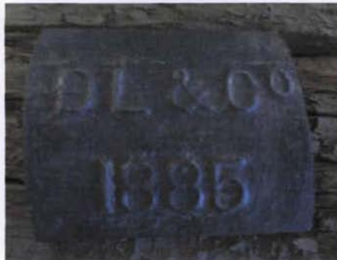
Photo 2: Manufacturer Plate on Wooden Pipe
