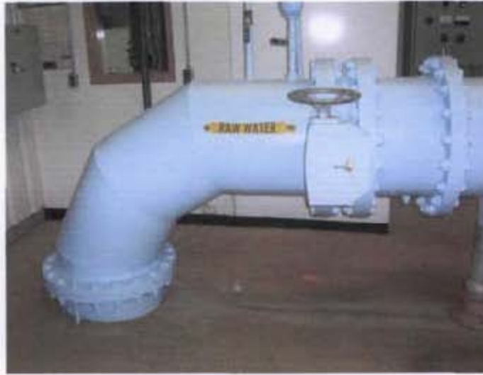
Photo 3: Water In-take to the Air Strippers
