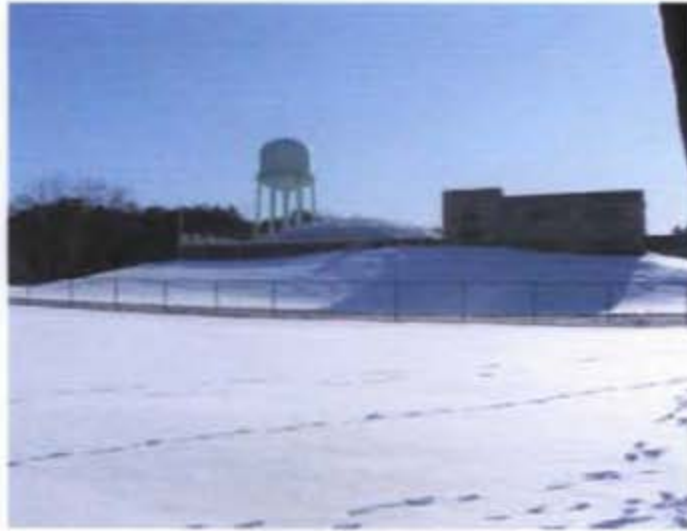
Photo 9: Water Treatment Plant
