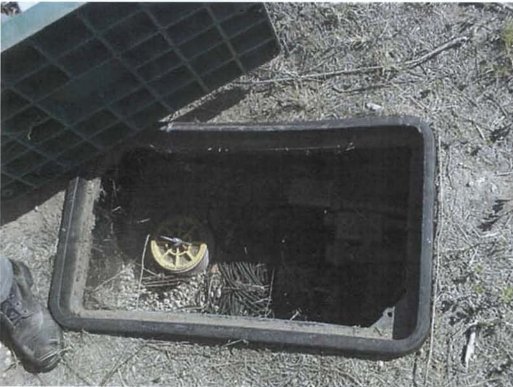
Photograph No. 8 Description: Monitoring well TW-6C
