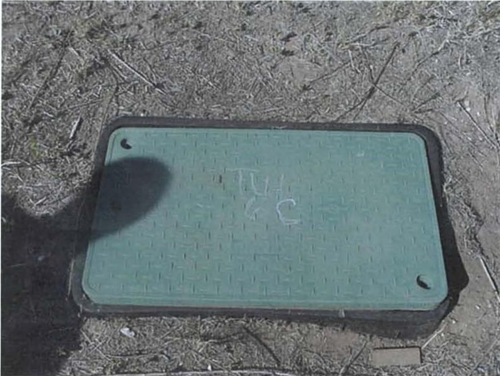
Photograph No. 7 Description: Monitoring well TW-6C
