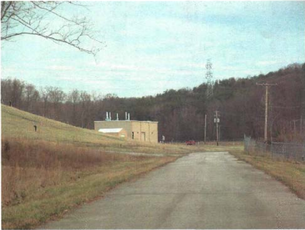
Photo 3- Inside Gate: looking toward leachate treatment facility; OU2 to left of structure, adjacent property and stream to right of photographer
