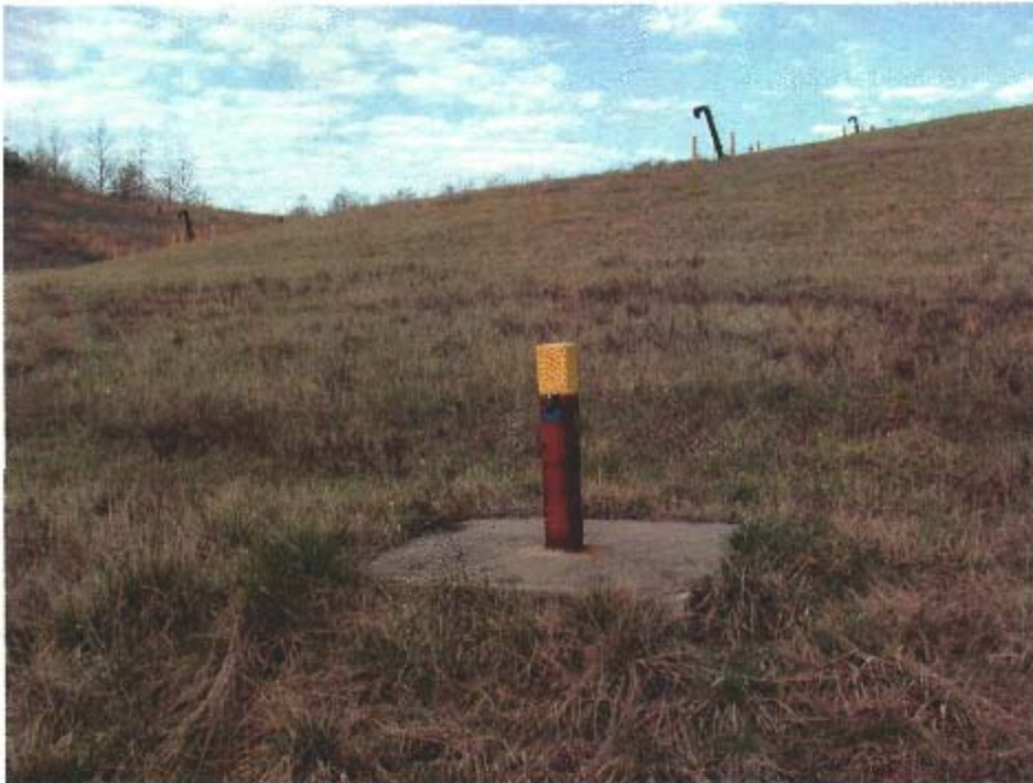
Photo 7- Typical Monitoring Well Installation
