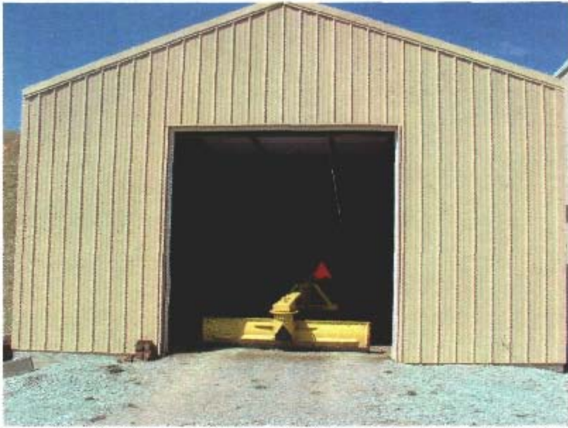
Photo 5- Storage for Maintenance Equipment: Adjacent to Leachate Treatment Structure
