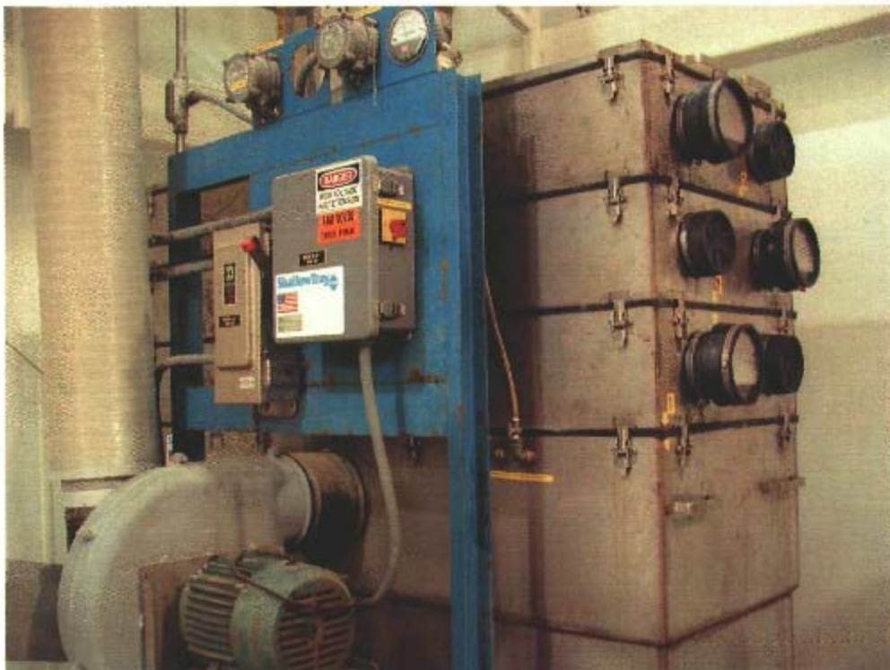
Photo 34- Package Low Profile Air Stripper (R-4-1)
