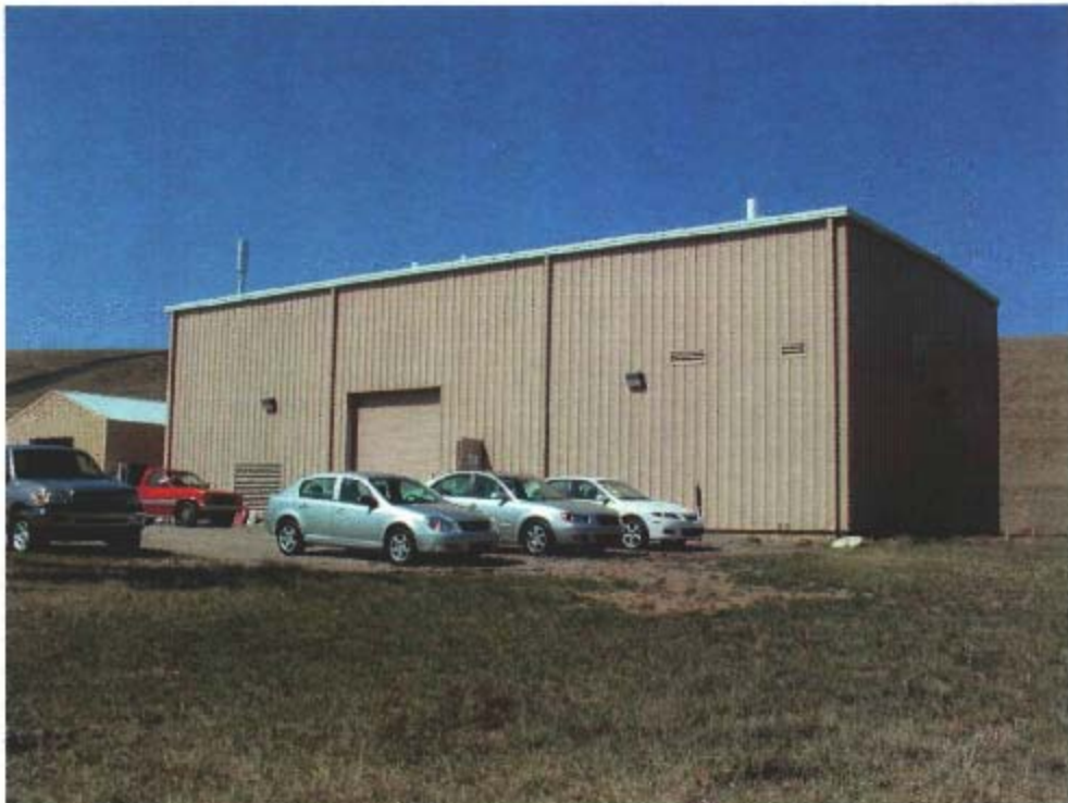
Photo 4- Leachate Treatment Facility
