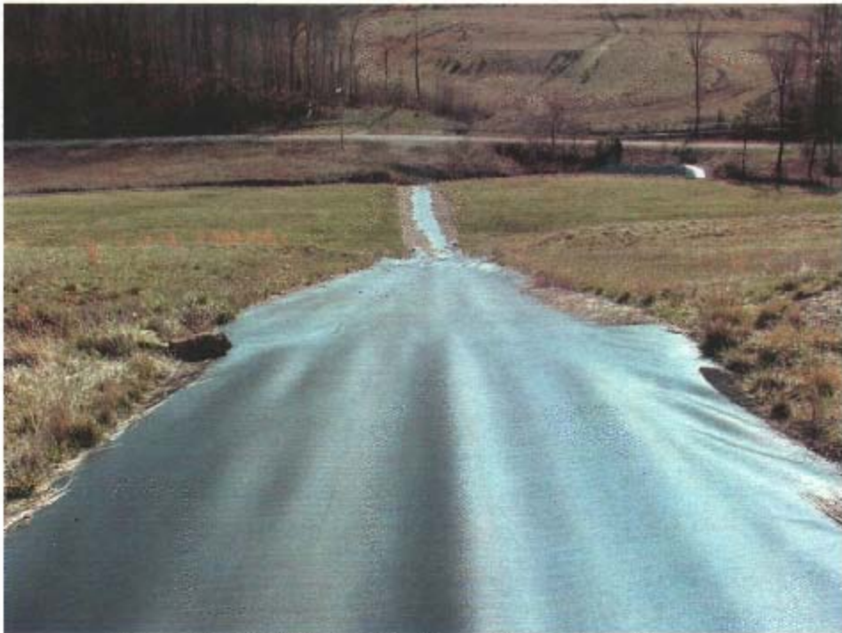
Photo 16- OU2 Typical Letdown Channel, looking east
