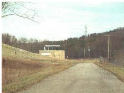
Leachate Treatment Plant
