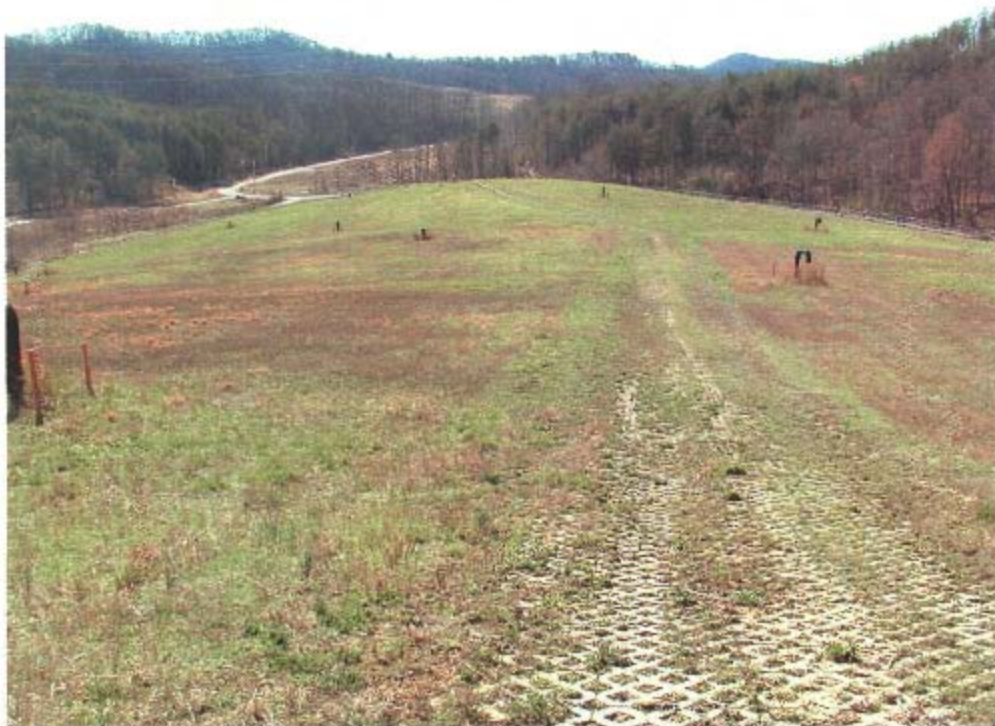
Photo 24- View Across OUI: Retaining wall to left of photographer, looking south.
