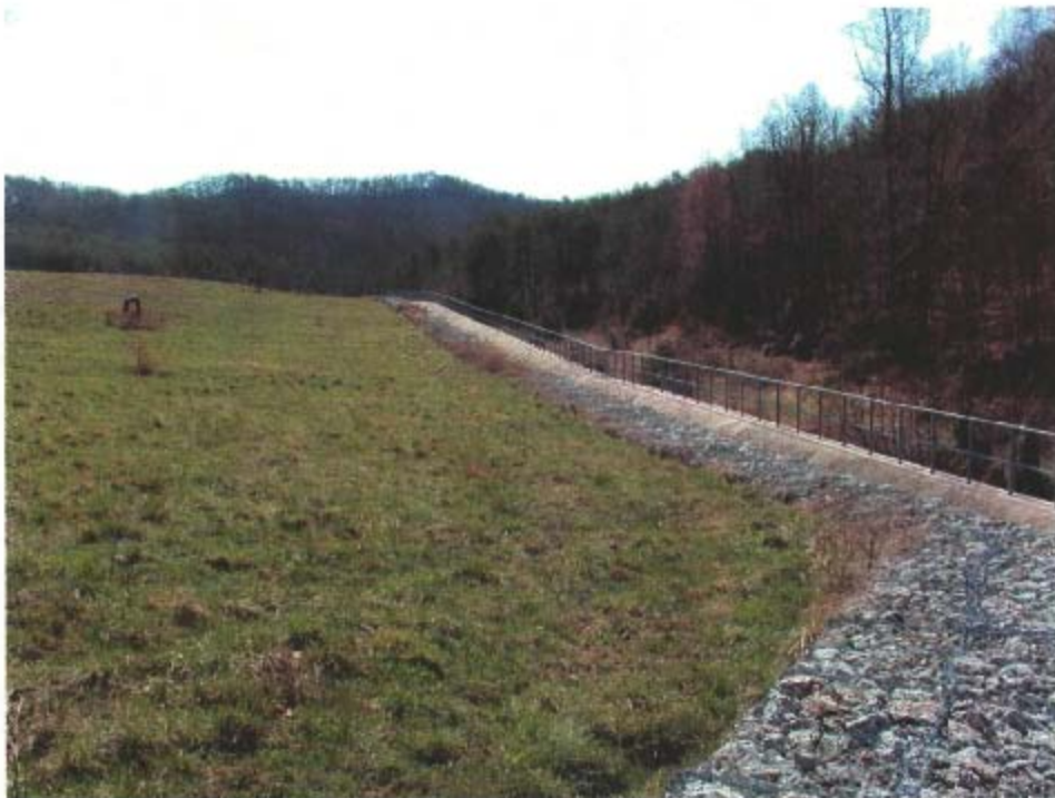
Photo 26- OU1 Western Boundary, looking south.
