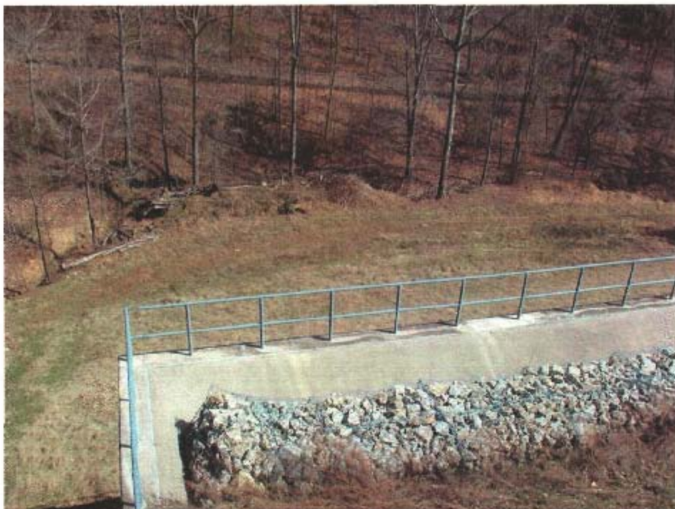
Photo 22- OUI: view down from top of retaining wall
