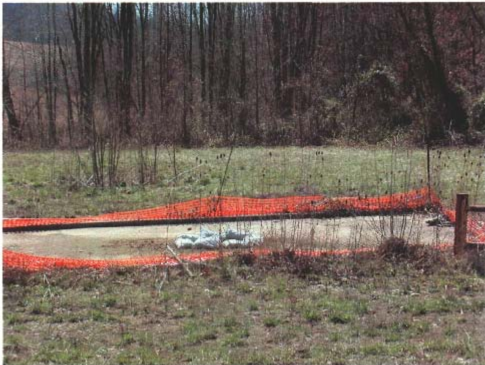
Photo 27- Sandbags protecting drain from debris at southernmost corner of OU1.
