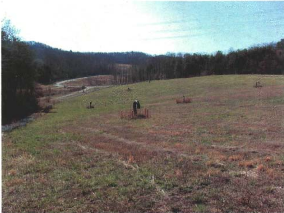
Photo 23- View Across OUI: Retaining wall to left of photographer, looking south.
