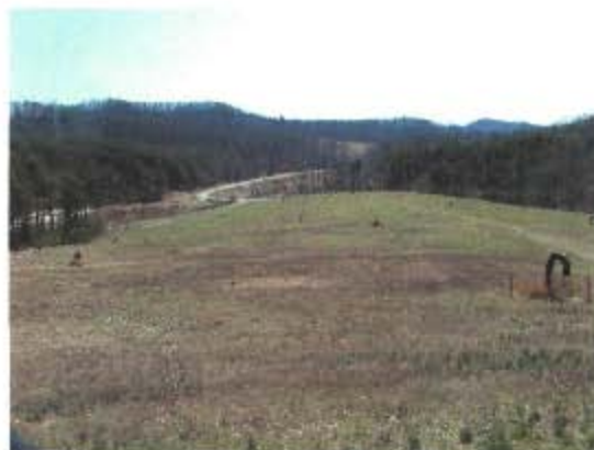
View Across OU1 Landfill Cap
