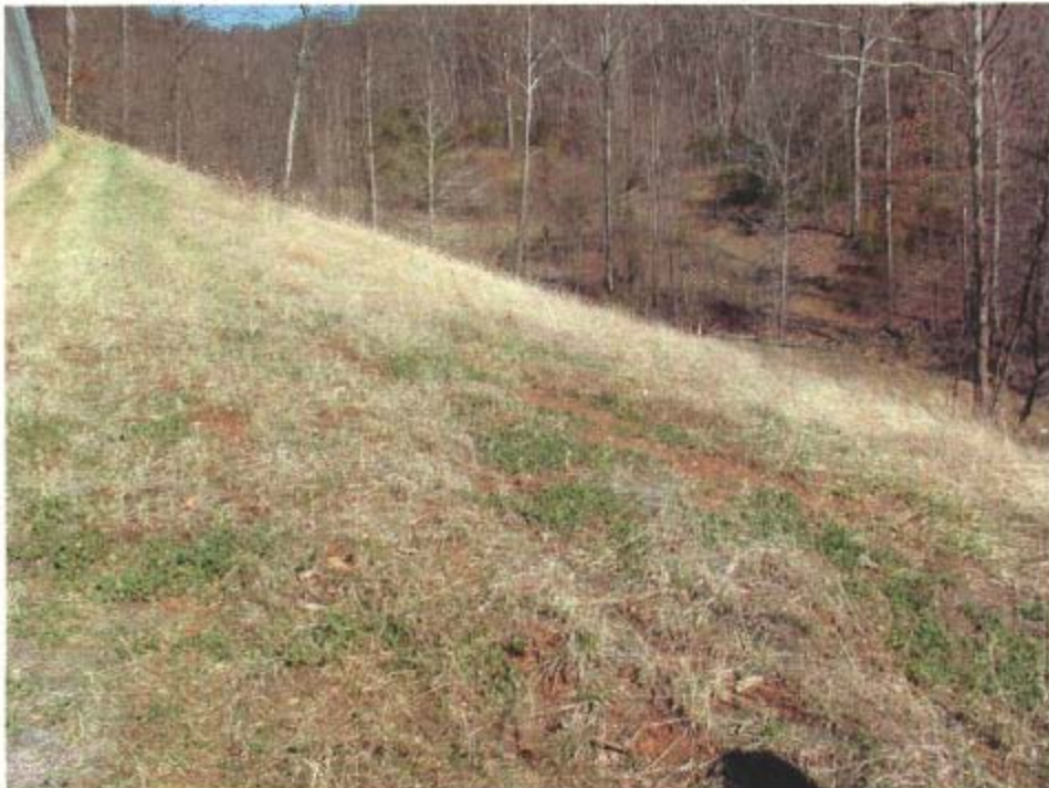
Photo 20- OUI Slope Near Retaining Wall
