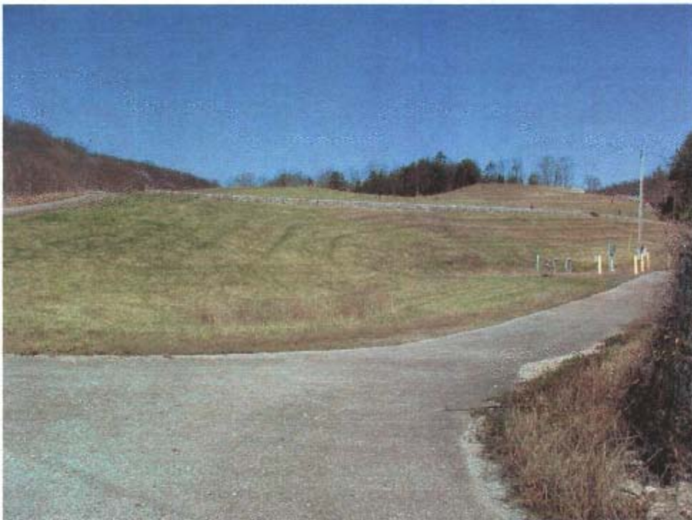
Photo 18- Base of OU1, looking northwest
