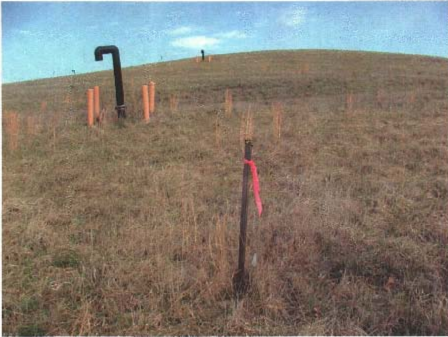
Photo 9- OU2: Marker for elevation monument (foreground), and gas vents (back)
