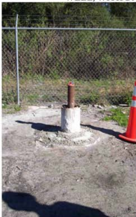
PHOTOGRAPH 12. INTERMEDIATE AQUIFER MONITORING WELL, WITH DNAPL, KOPPERS, 1 FEB 06
