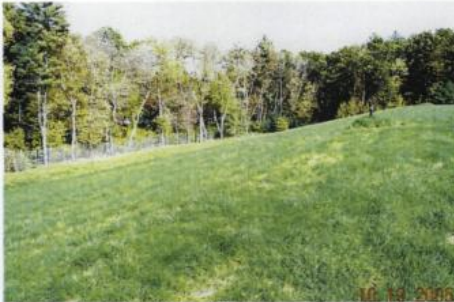
Photograph 1 – Sudbury Landfill looking northeast from the crest.
