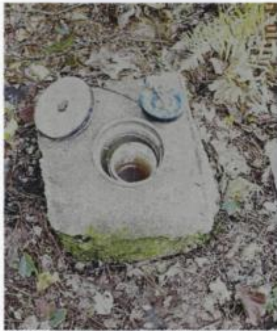
Photograph 4 – Example Photo of Damaged Wells Between the Landfill and the Assabet River.
