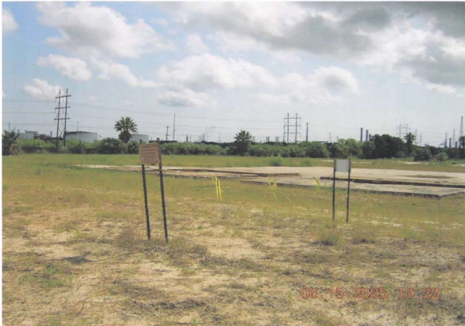
Photo 3: OU1: Concrete floor slab from former building. Signs mark the location of the slurry wall.
