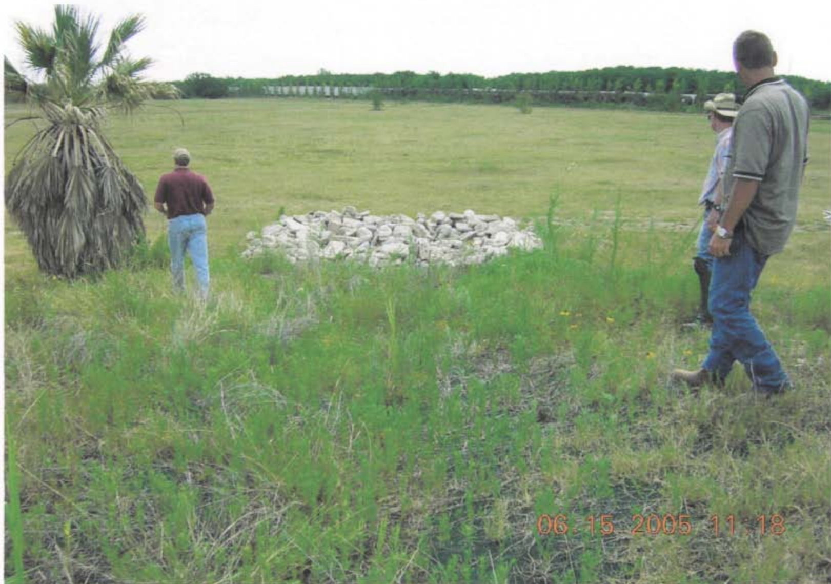
Photo 18: OU1: NORM Disposal Cell letdown channel showing rip-rap.
