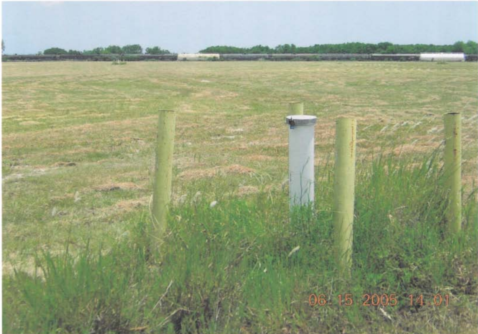
Photo 35: OU2: Site groundwater monitoring well. ID tags and locks were missing (facing east).
