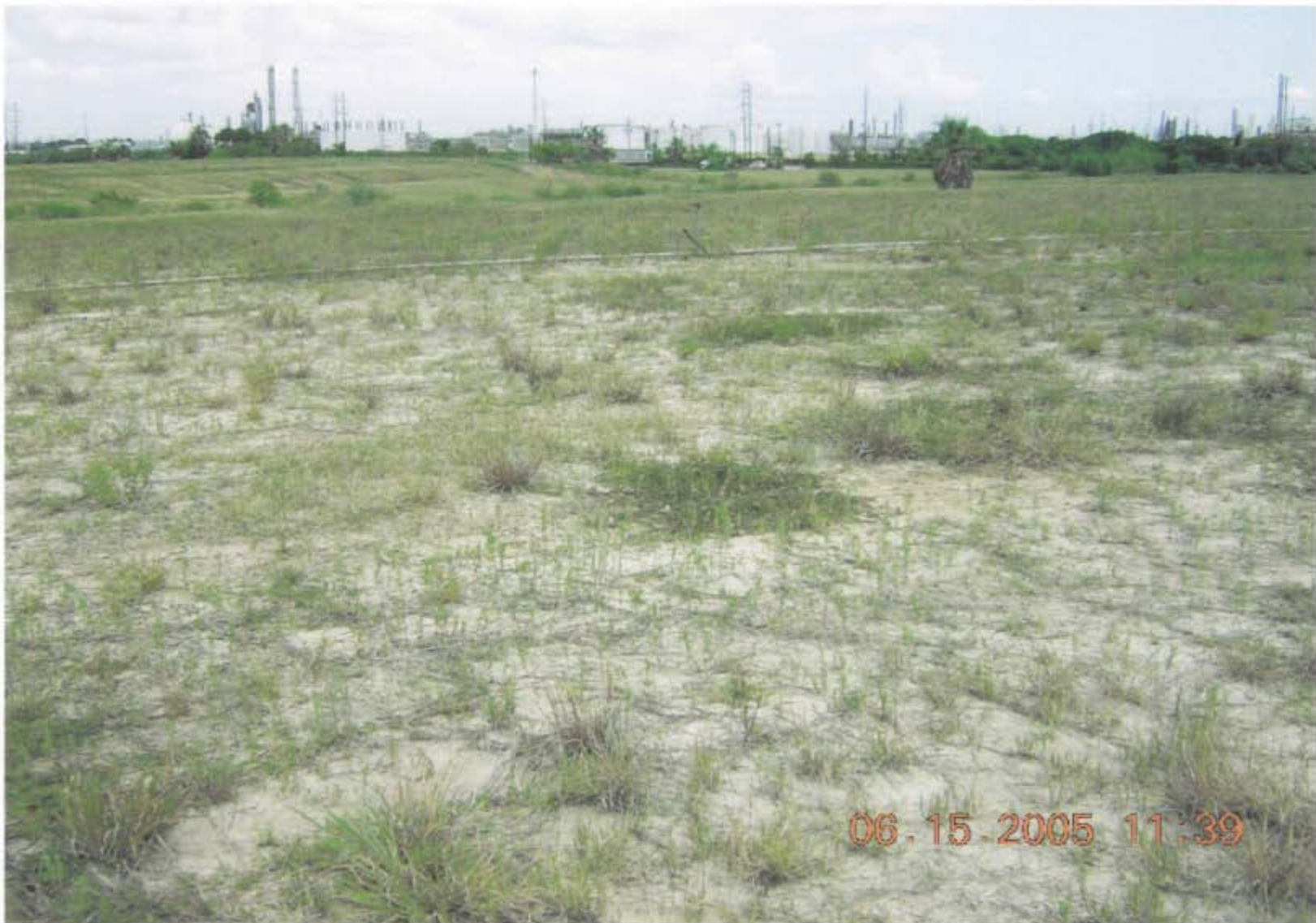
Photo 27: OU1: Top of the Consolidation Cell.
