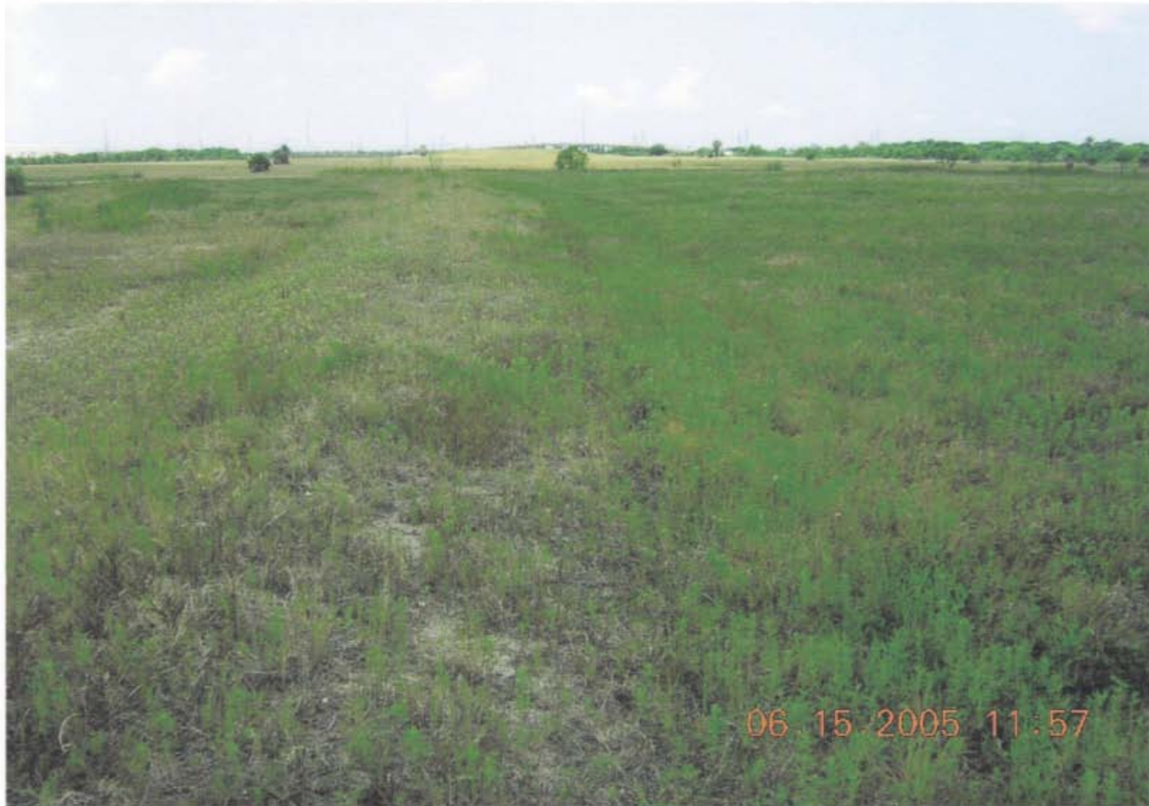
Photo 32: OU1: Facing south across west slope of Pond 7 cover.
