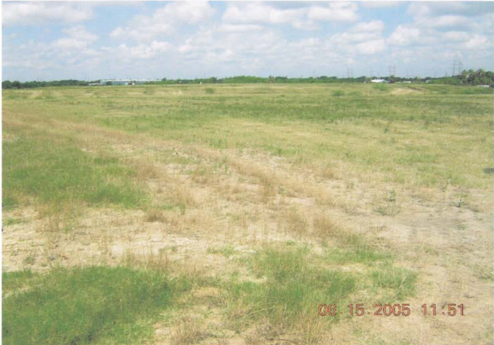
Photo 29: OU1: Facing northwest across northeast side of Consolidation Cell.
