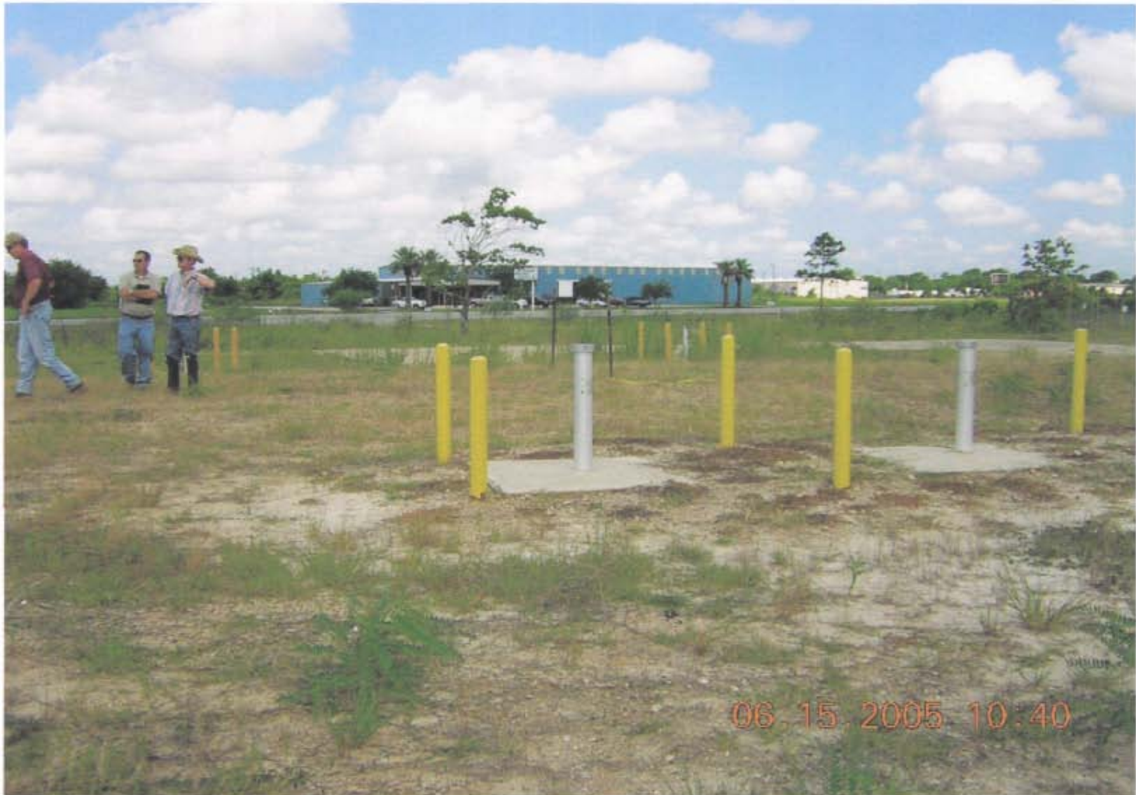
Photo 5: OU1: Groundwater monitoring wells on west side of site. All ID tags and locks are in place.
