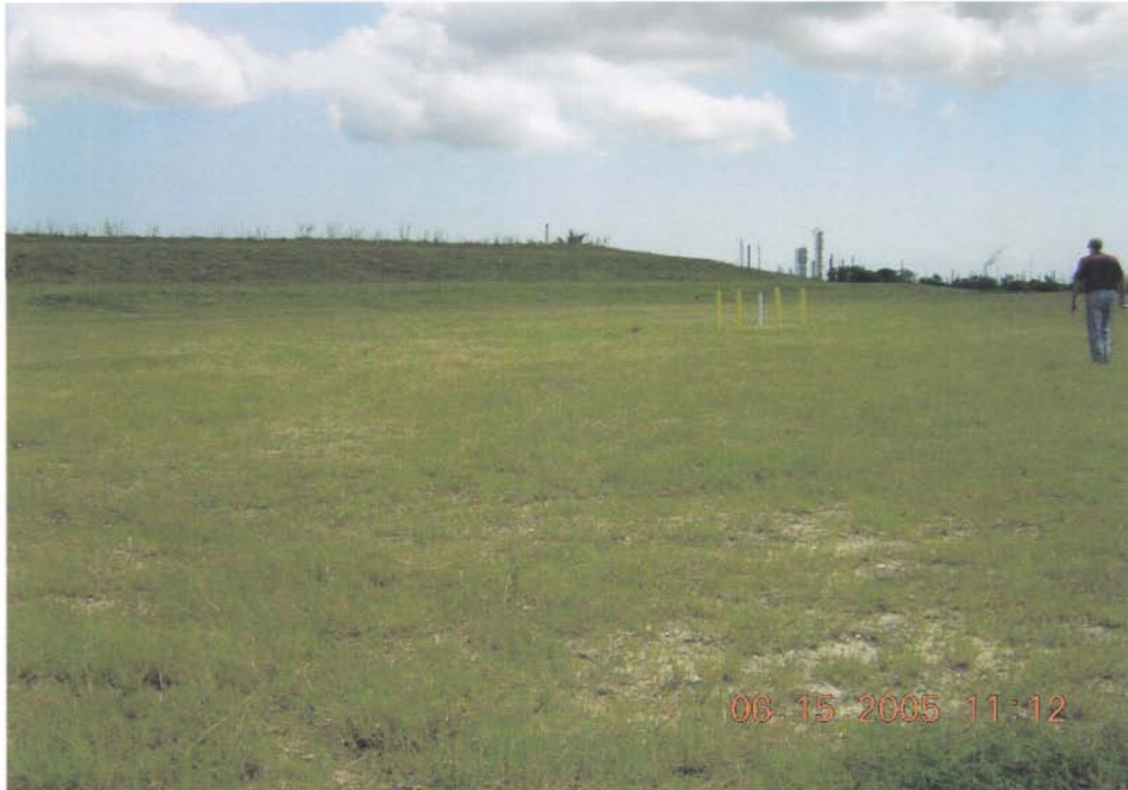
Photo 14: OU1: NORM disposal cell.
