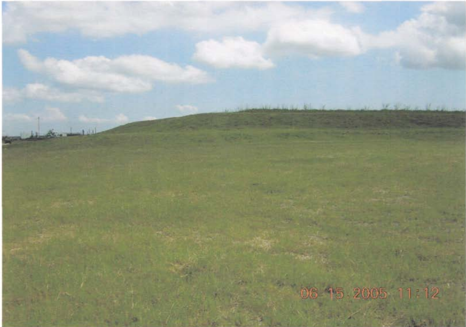
Photo 13: OU1: NORM disposal cell.
