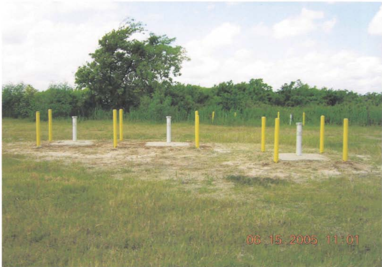
Photo 10: OU1: Site groundwater monitoring wells. All ID tags and locks are in place.
