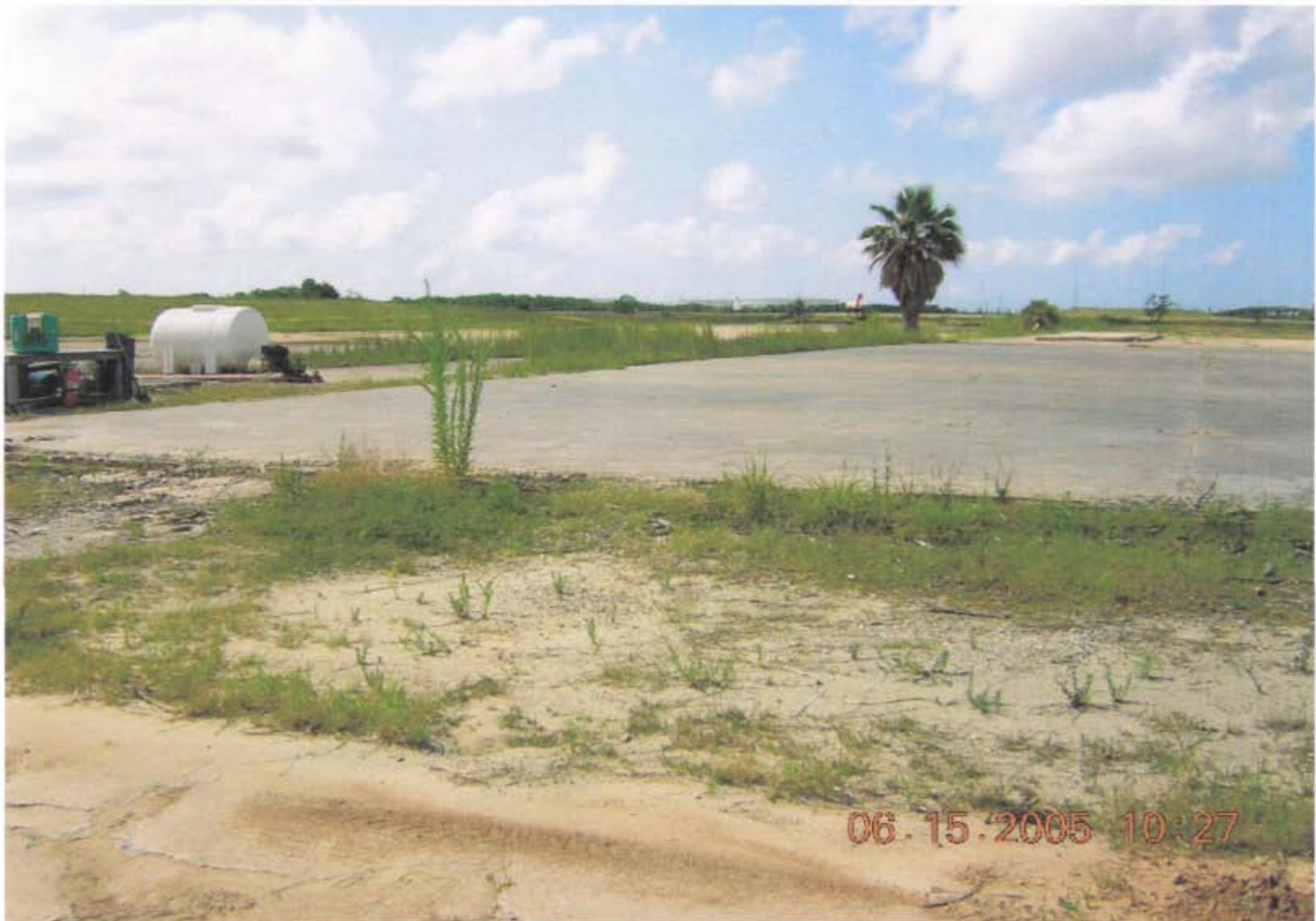
Photo 2: OU1: Concrete floor slab from former building.
