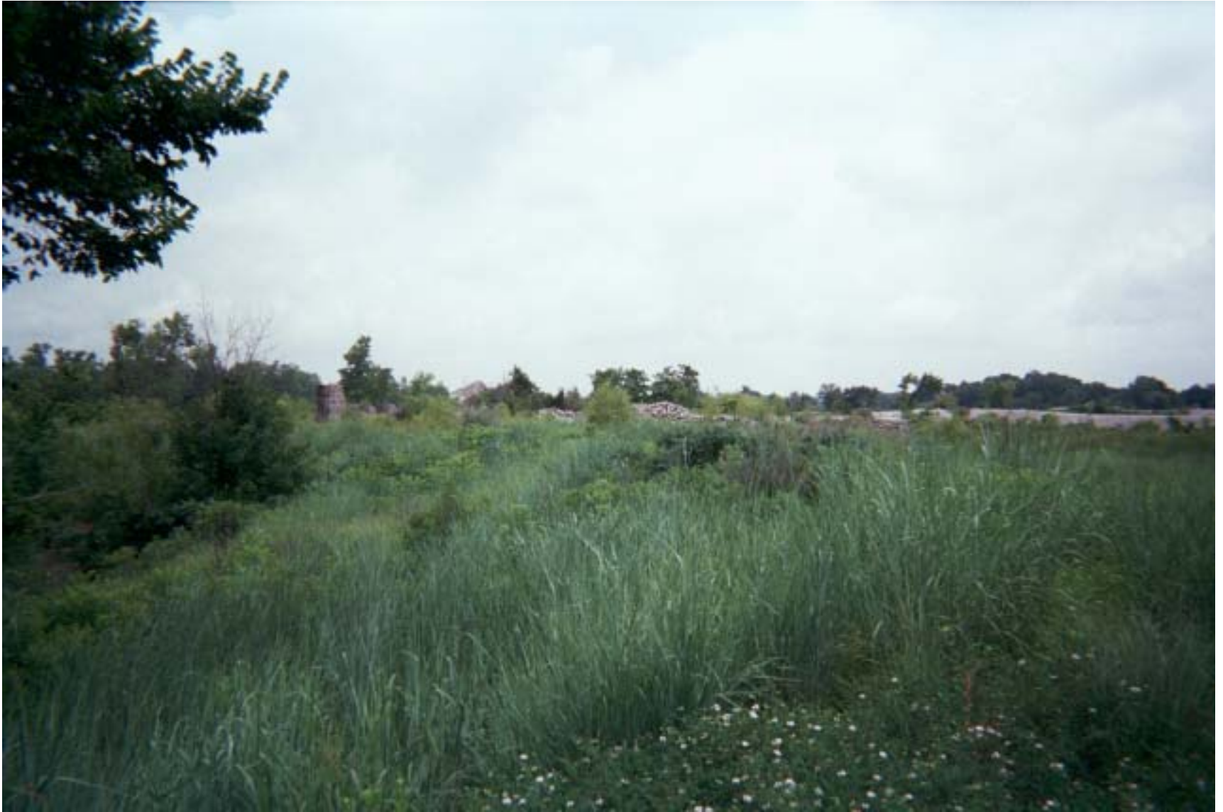
Photo 62: View of diversion dike at the Big John Mine site, located in Kansas. The subsidence feature is located to the left of this view.
