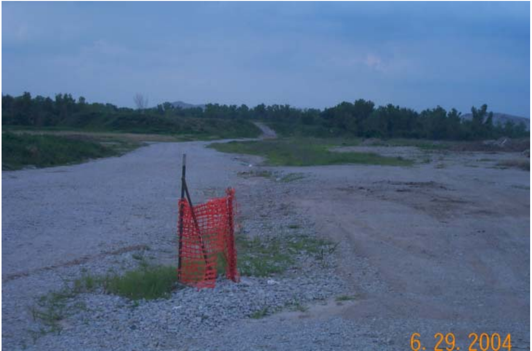
Photo 25: View of repository on E40 Road facing east.
