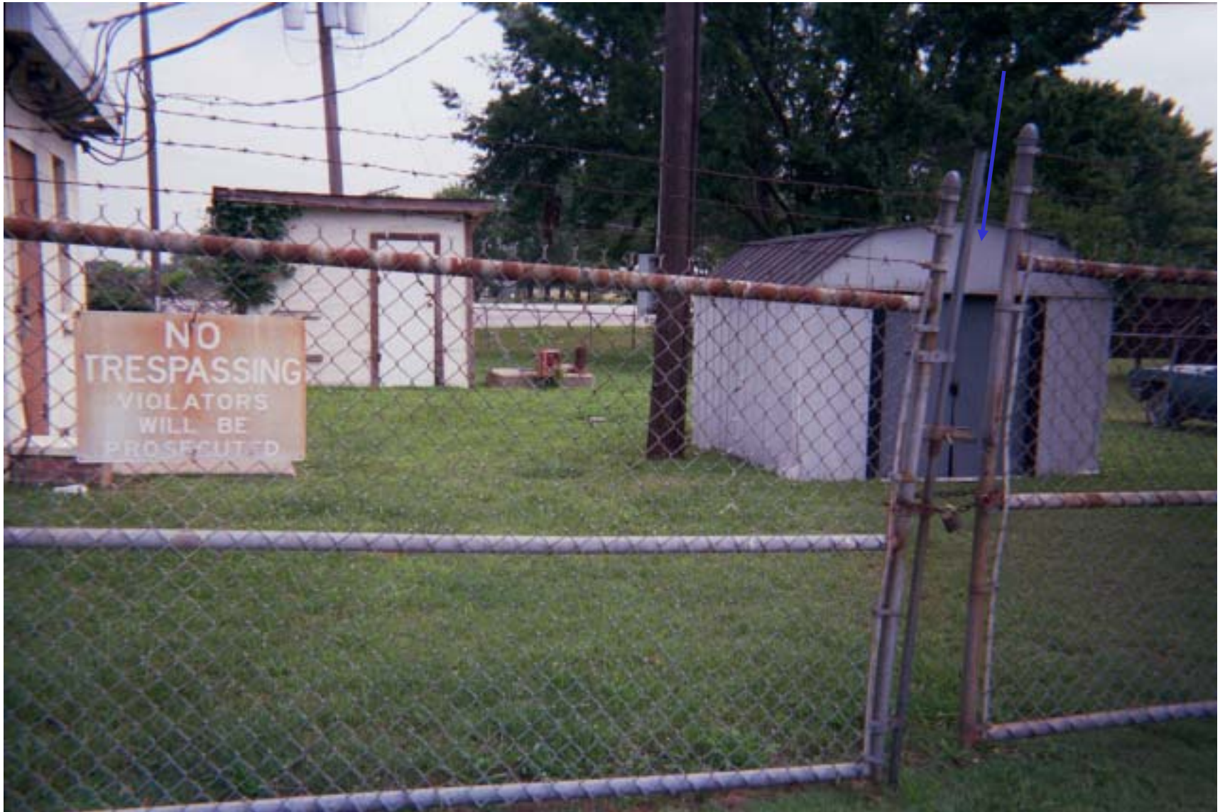
Photo 53: View of Quapaw #2 well location. Well is located inside shed at right (blue arrow).
