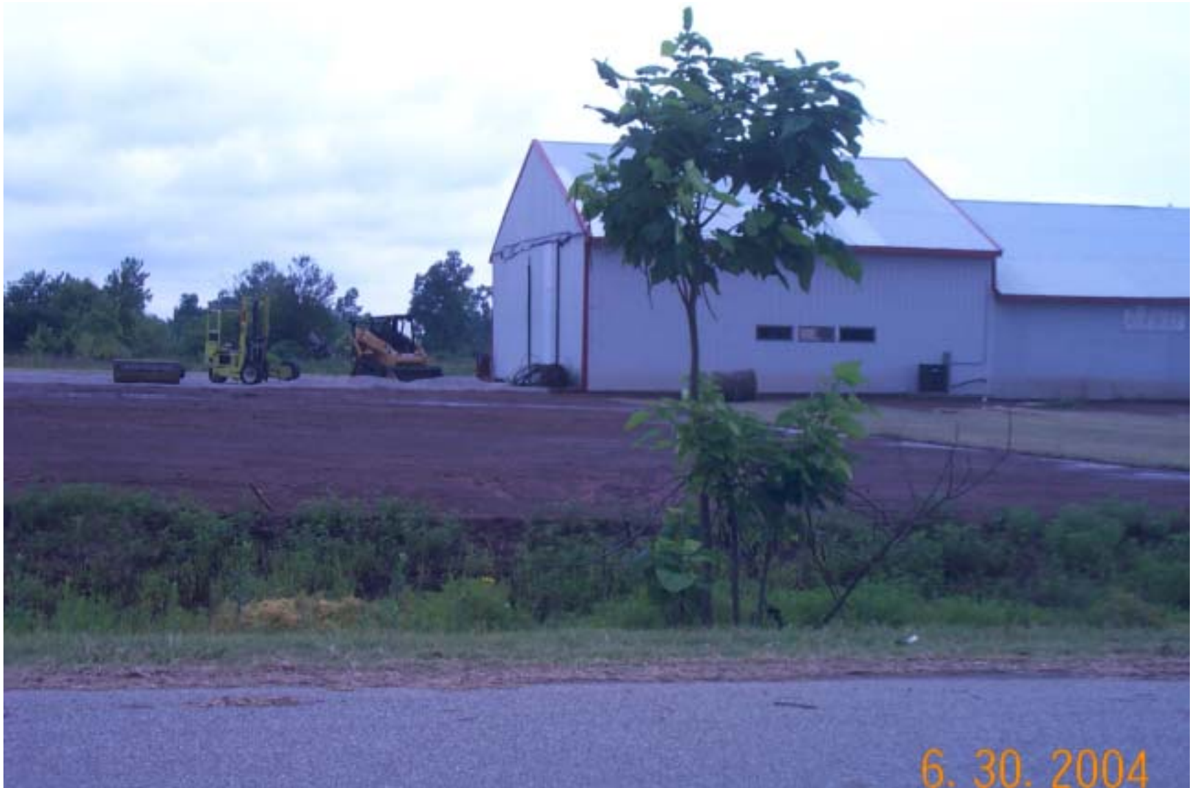
Photo 33: View of property in North Miami, Oklahoma. Construction was not complete at the time of the site inspection. Area in the foreground is where replacement sod has not yet been placed.
