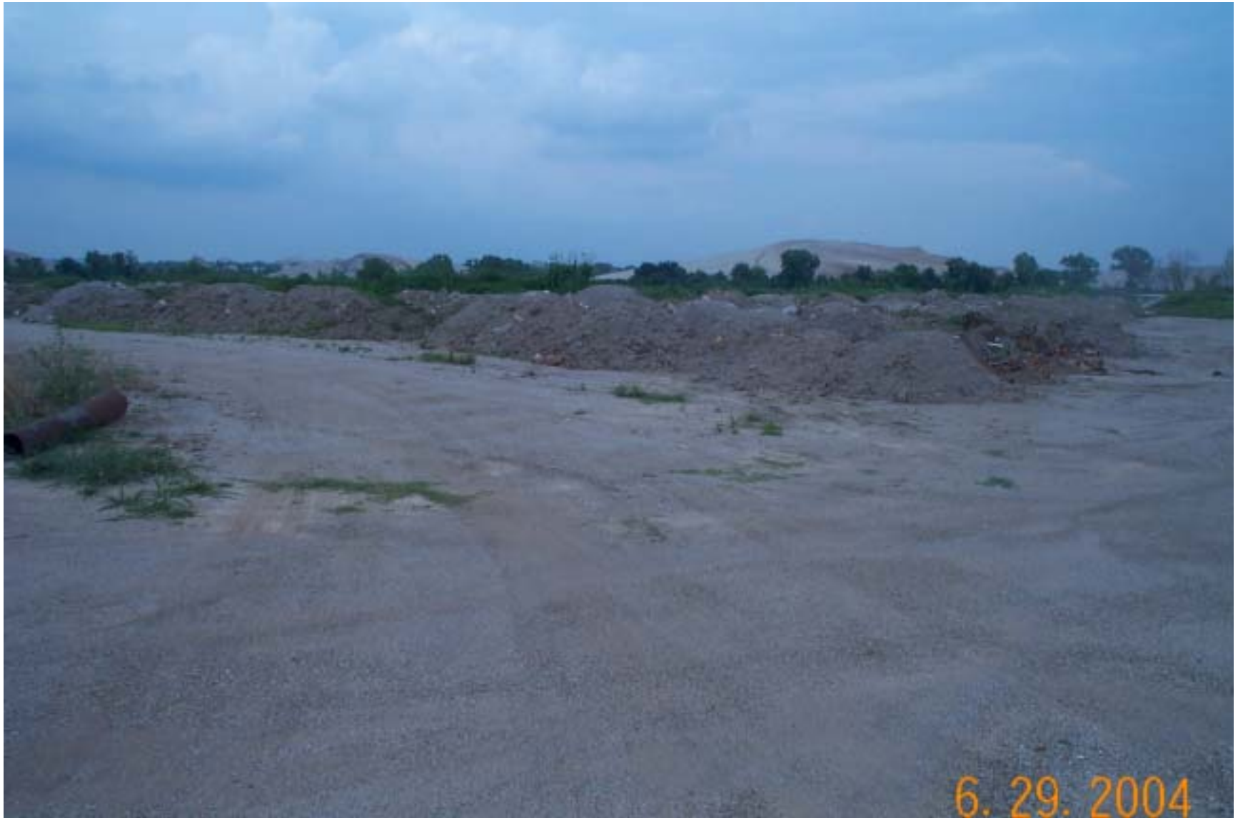
Photo 26: View of recently deposited soil at the repository on E40 Road. Lead contaminated soil from residential yards is used at the repository to fill in an old mill pond.
