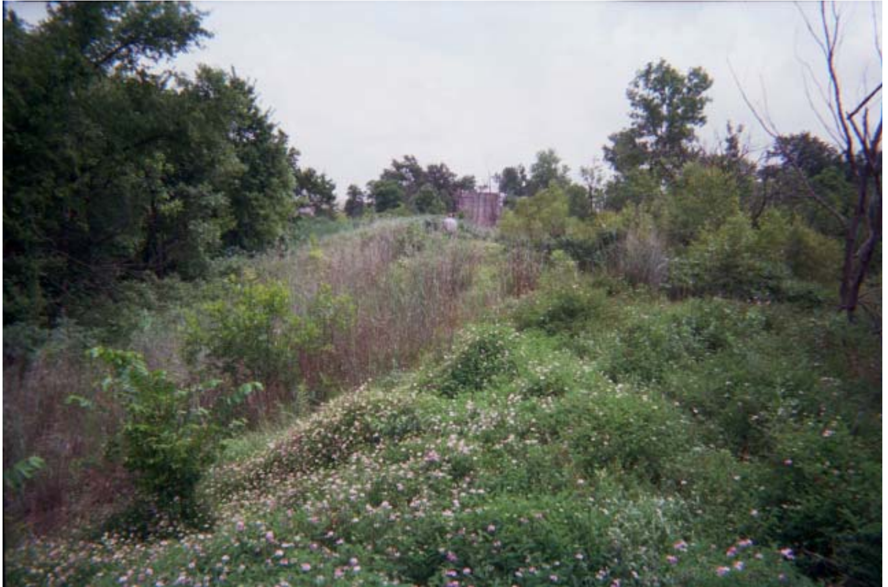
Photo 58: View of diversion dike at the Big John Mine site, located in Kansas.
