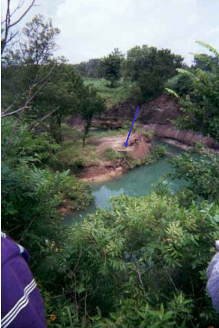
Photo 60: View inside subsidence at the Big John Mine site, located in Kansas. A diving board is visible in the center of the picture (at blue arrow). ODEQ noted that this location is frequented by swimmers.
