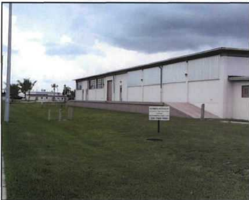
Photograph 8: Operable Unit 15 – Hazardous Waste Storage Building
