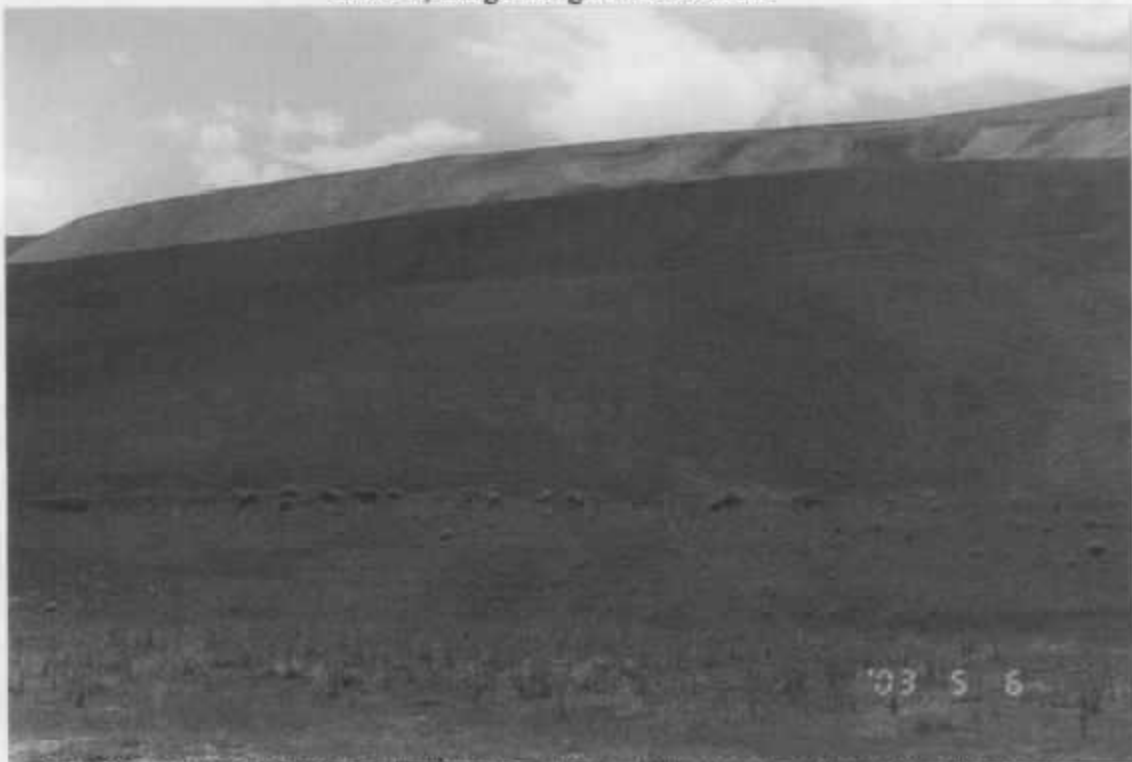
Relaxed Slope of Dumps where sludge, lime, soils mixed and used for the slope
