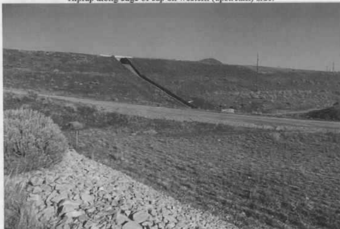
Large Bingham Reservoir Dam from tailings pond showing riprap on the upstream side
