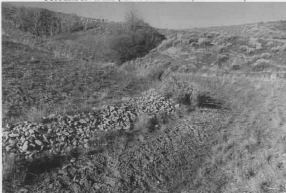
Riprap along edge of cap on western (upstream) side.
