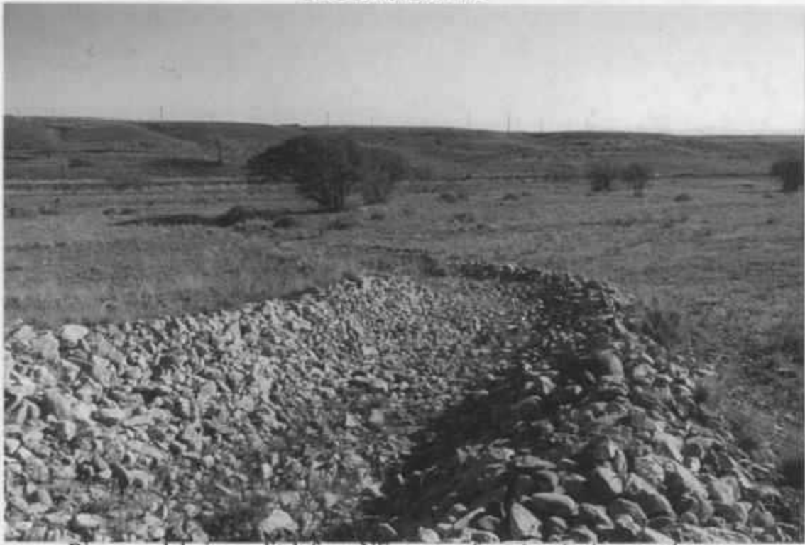
Riprap and drainage ditch from NE corner of cap to retention pond area
