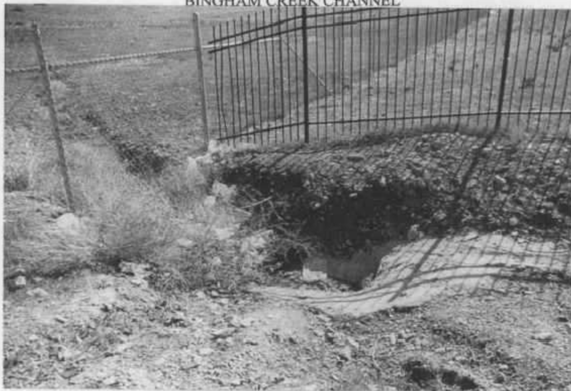
Ditch from highway and access road leading to erosion gully to Bingham Creek
