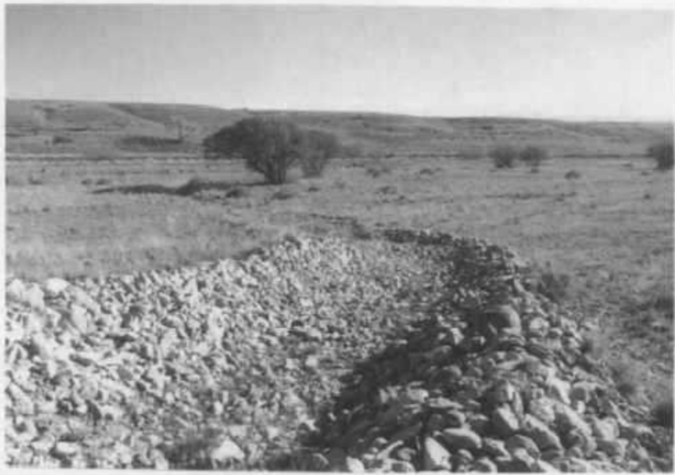
Figure 15: Drainage ditch with larger rip-rap lining
