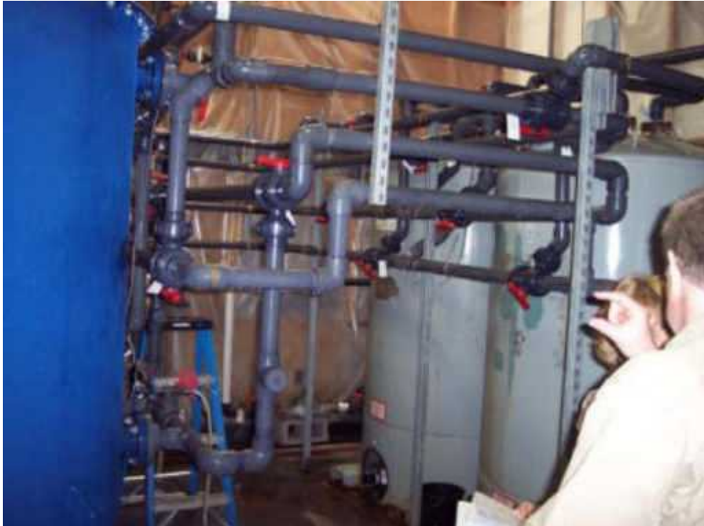
UniFirst Photo 8: Carbon Units
