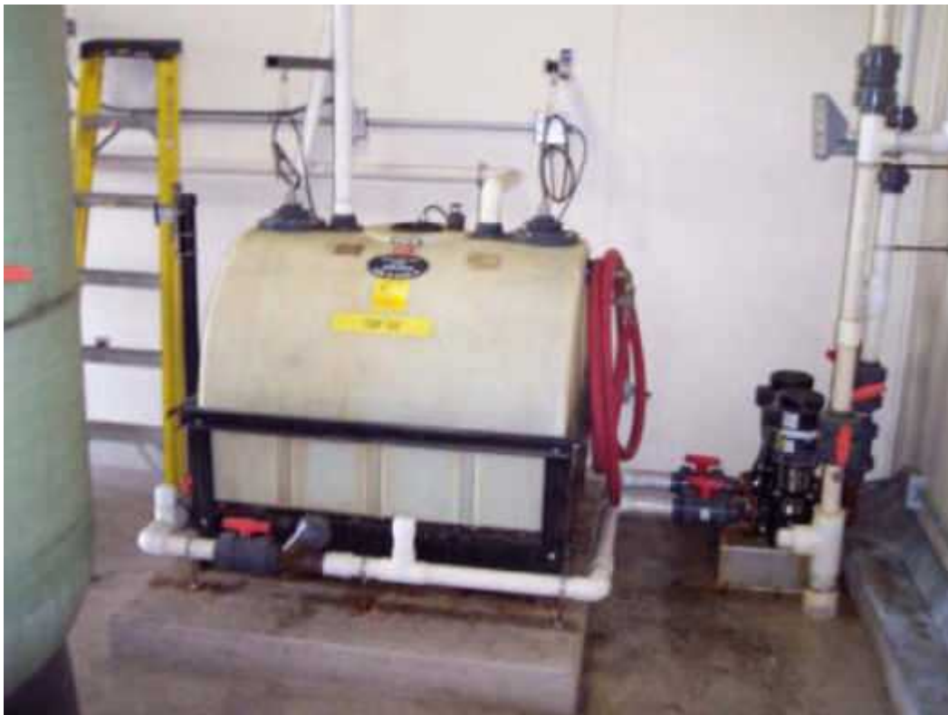
Grace Photo 4: Equalization Tank
