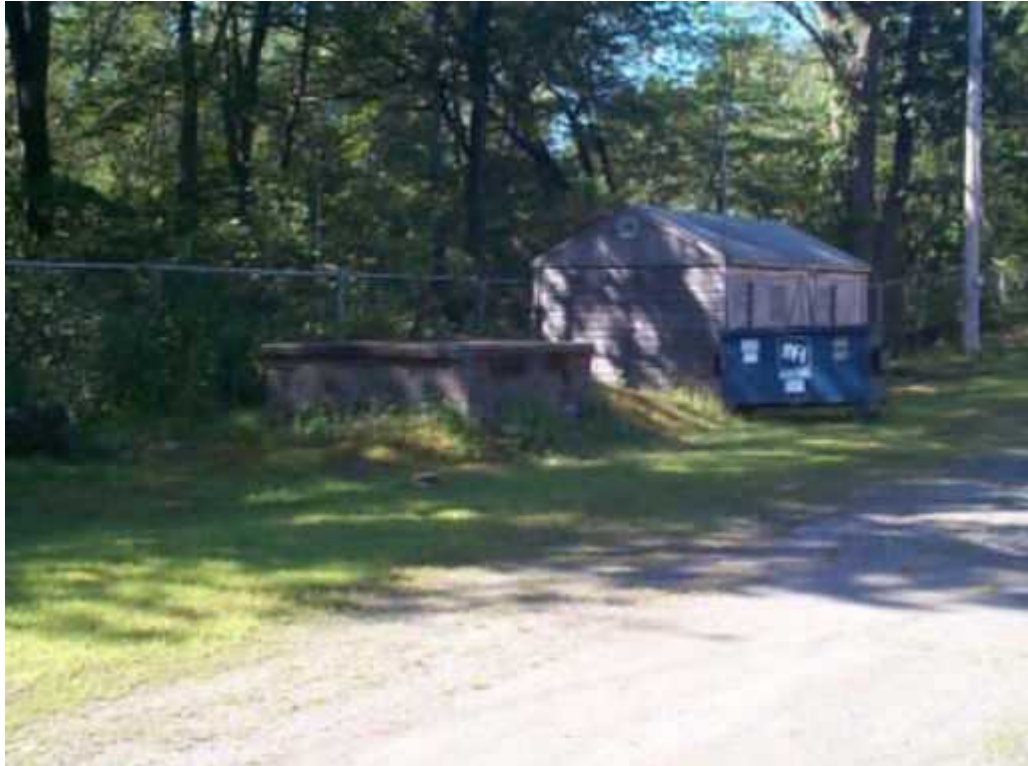
Wildwood Photo 1: Riley Well Enclosure and Storage Shed
