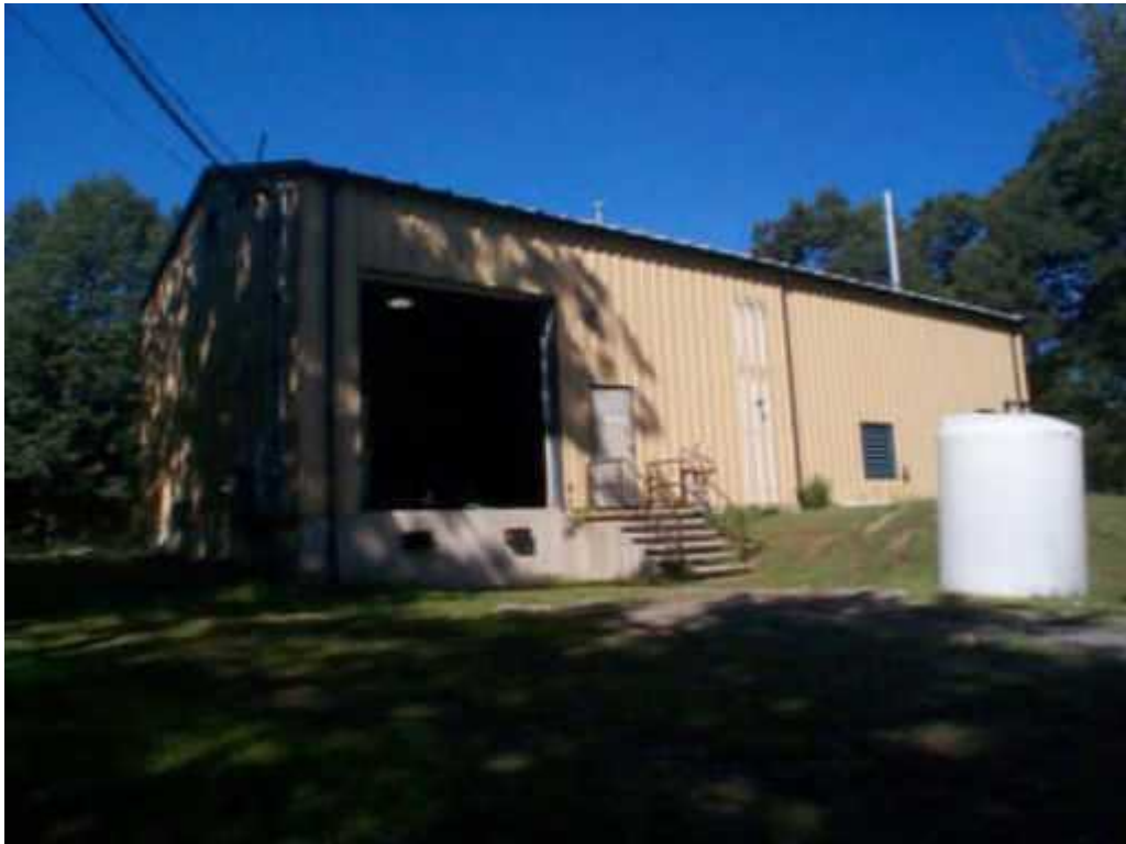
Wildwood Photo 2: Treatment Building
