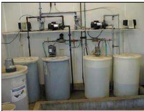
Photos 21 and 22: Lidgerwood Water Treatment Plant, Permanganate and Fluoride Chemical Feed
