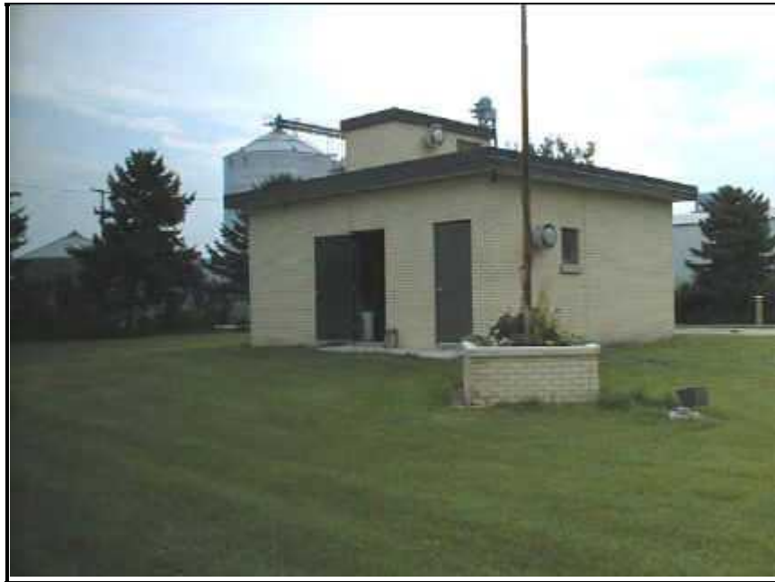
Photo 1: Wyndmere Water Treatment Plant Building
