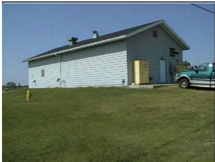
Photo 16: Lidgerwood Water Treatment Plant Building
