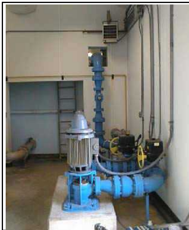
Photo 23: Lidgerwood Water Treatment Plant
