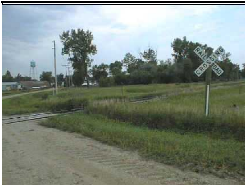
Photo 7: Clay Cap in Wyndmere that covers area which arsenic trioxide was mixed. Cap is located between the railroad tracks, power lines, and trees.
