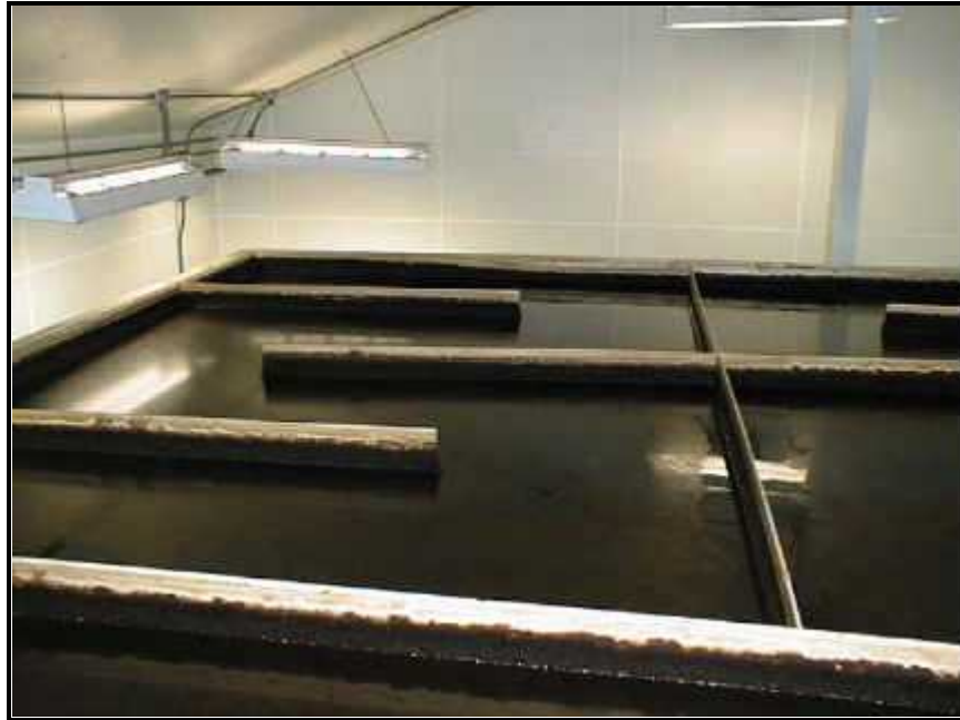
Photo 19: Lidgerwood Water Treatment Plant
