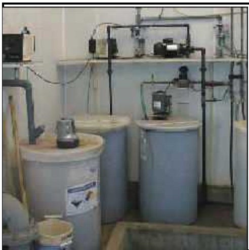
Photos 21 and 22: Lidgerwood Water Treatment Plant, Permanganate and Fluoride Chemical Feed
