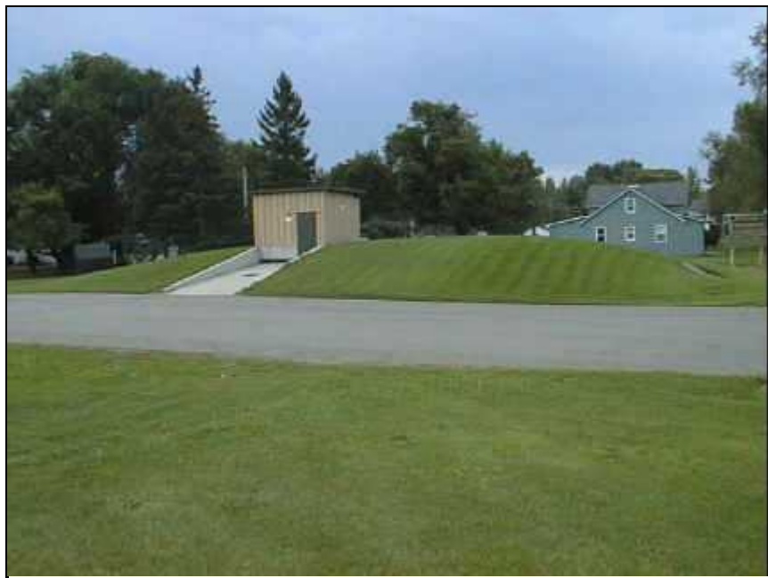
Photo 2: Wyndmere Underground Water Storage Tank
