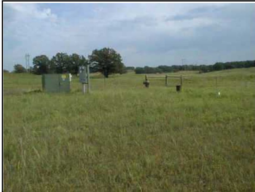
Photo 9: Underground Water Storage Tank Southeast Water Rural Water System
