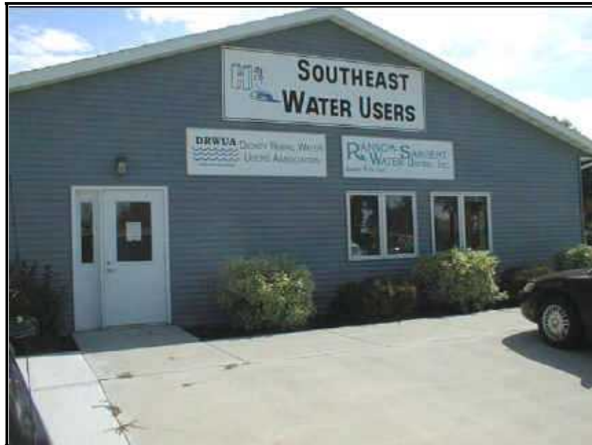
Photo 15: Southeast Water Rural Water System office building
