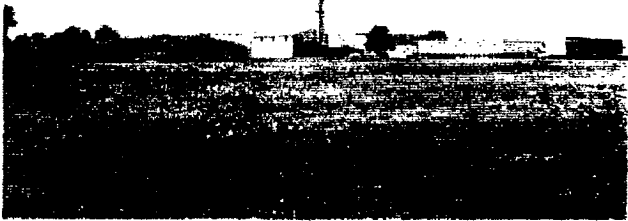
FIGURE 5. GWEX TREATMENT PLANT
