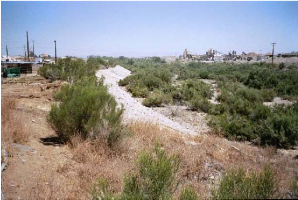
View of Bank Stabilization at RW-02
