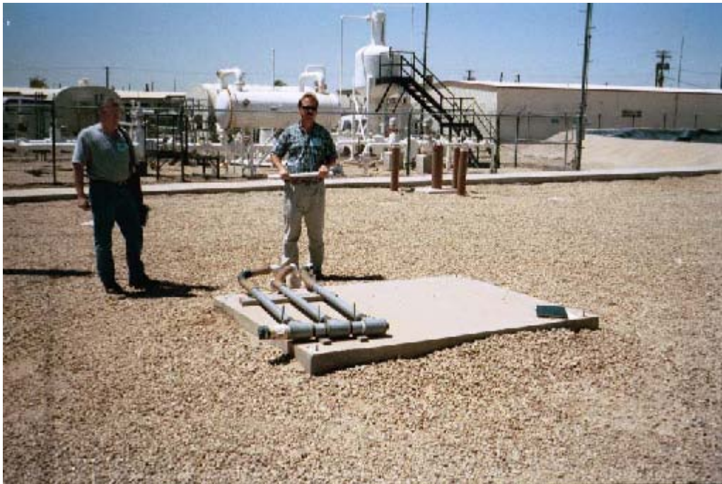
SS-42 pad where SVE pad was
