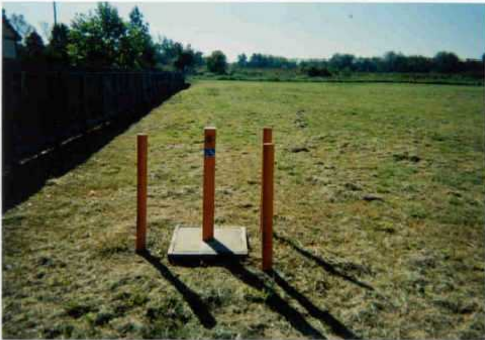
14) Monitoring Well AB-21D
