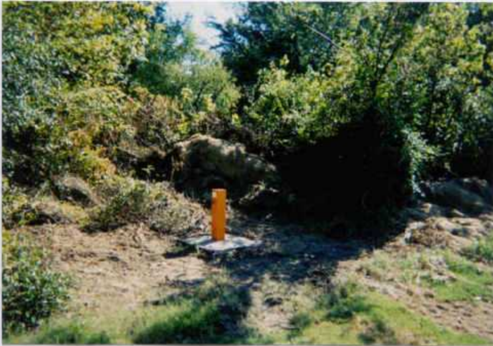
11) Monitoring Well AB-17D
