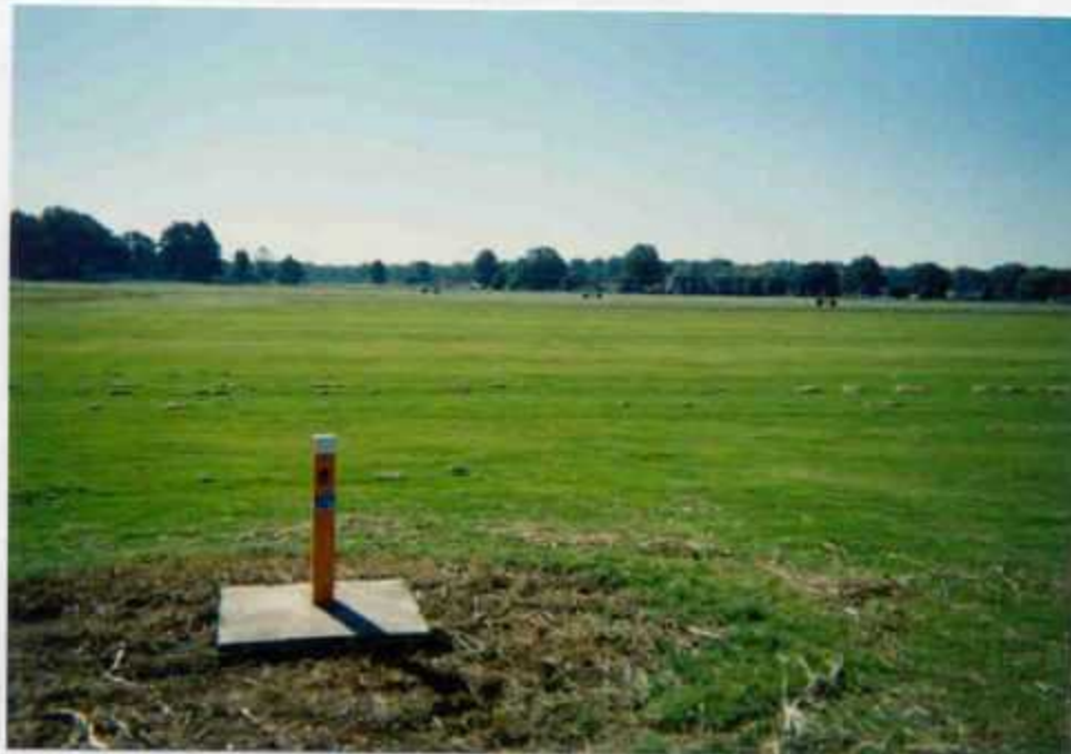
10) Monitoring Well AB-15D
