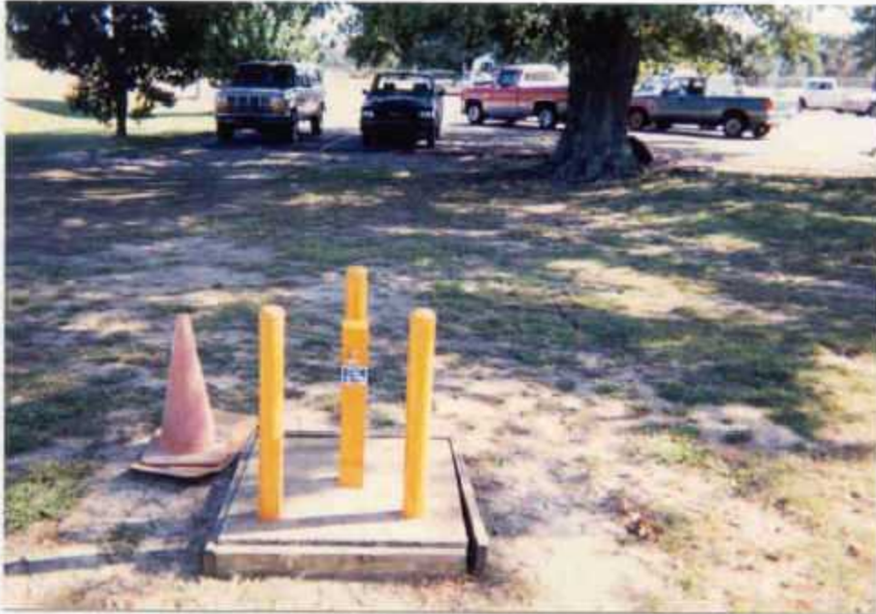
7) Monitoring Well AB-8D
