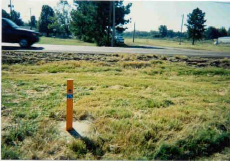
9) Monitoring Well AB-13D
