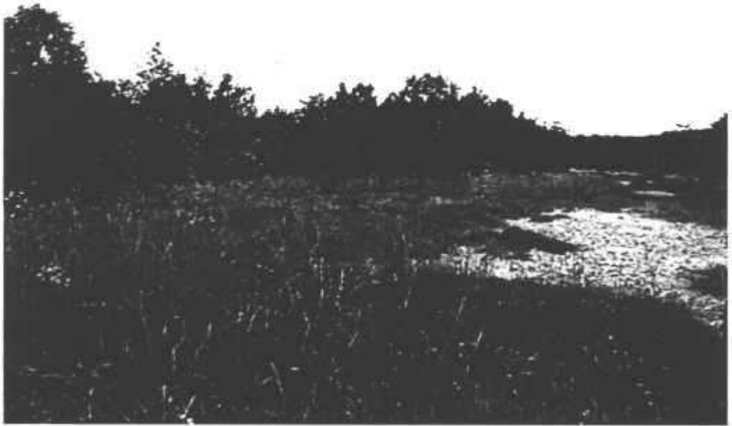
Photograph: Landfill cover near LW-2 Project Name: Cedartown Municipal Landfill Superfund Site
