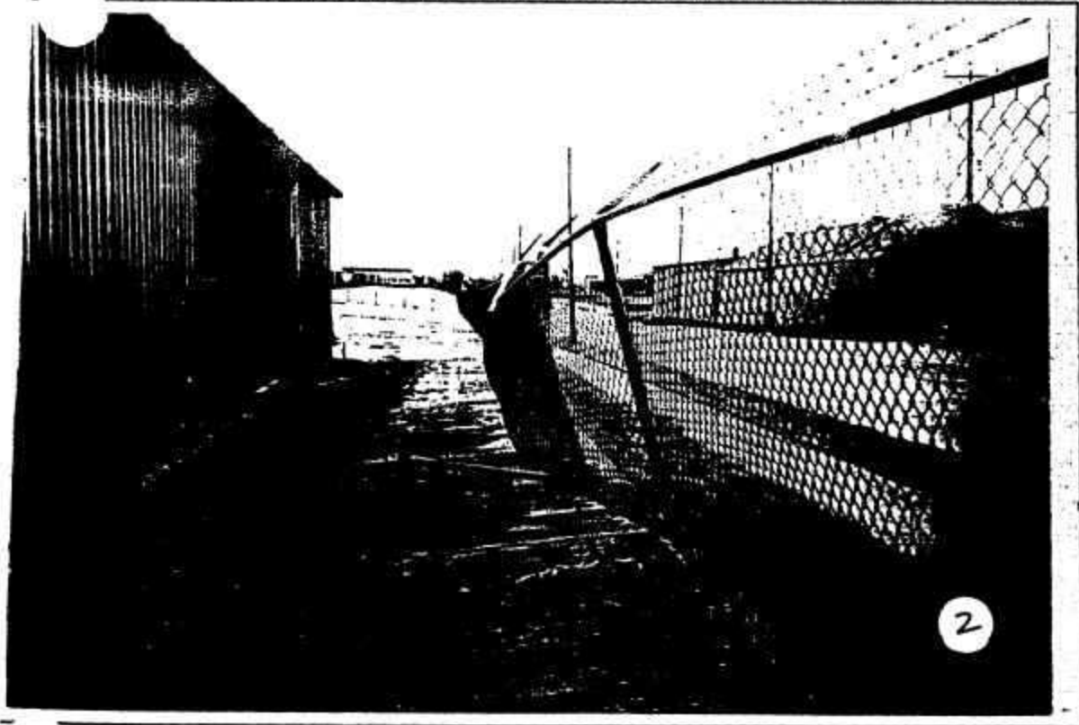
Photo #2 - (13:20 am) - Two of the fence posts were noted damaged and the chain link fence had been stretched but not penetrated as shown above. Photo taken just inside the west entrance gate facing south.
