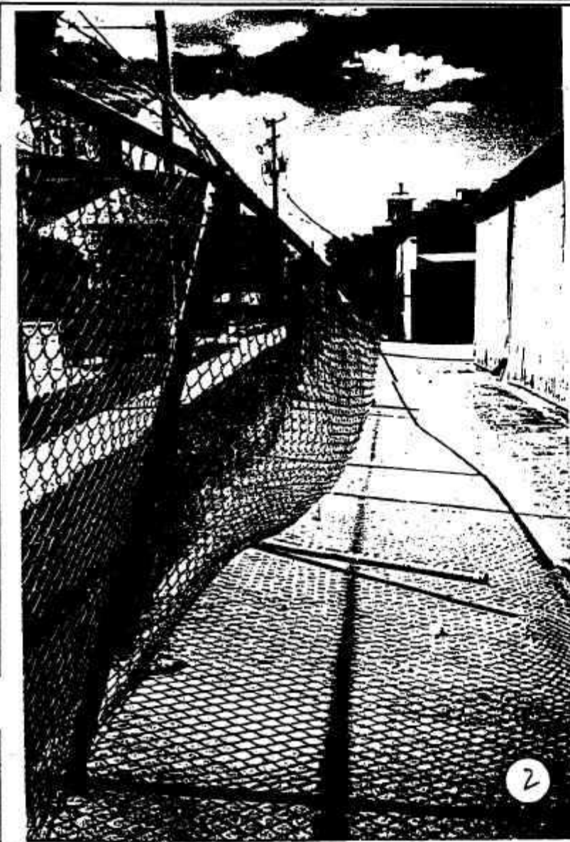
Photo #1 - The damaged portion of the perimeter fence included approximately 20' located along the west side of the site as shown above. Photo taken facing south.
