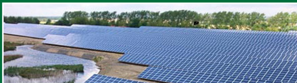
Photovoltaic arrays at Leipziger Land Solar Power Plant (source: GEOSOL)
