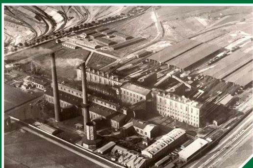
Former Borna briquette plant (source: GEOSOL)
