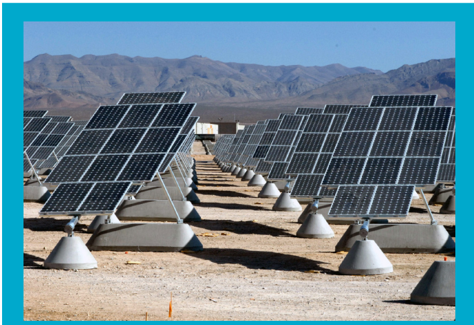
Tilted toward the south, each set of solar panels at the Nellis Air Force Base solar power plant rotates on a swivel to track the sun from east to west. (Source: US Air Force)
