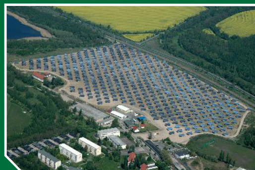
Today, 3.4 MW PV array (source: GEOSOL)
