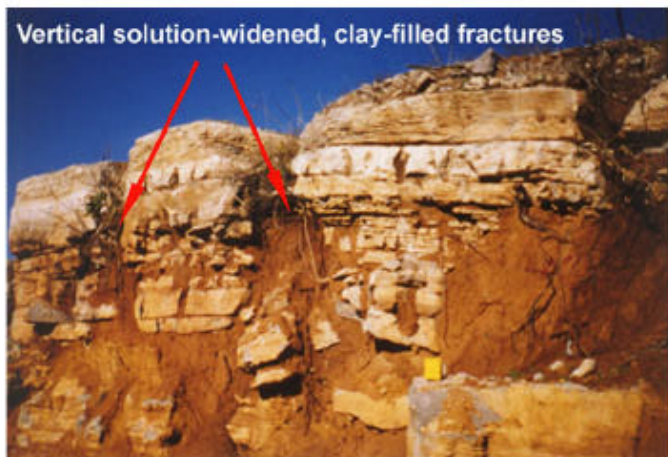
Vertical solution-widened clay-filled fractures, seen at a road cut in the area.
