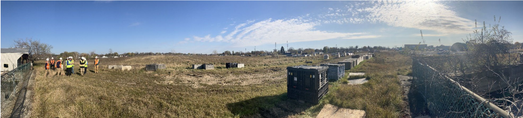
View of the FPS area that will be capped once OU1 remediation is complete.
