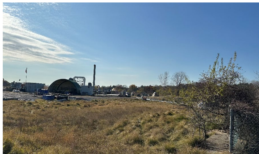
In situ soil treatment operations.
