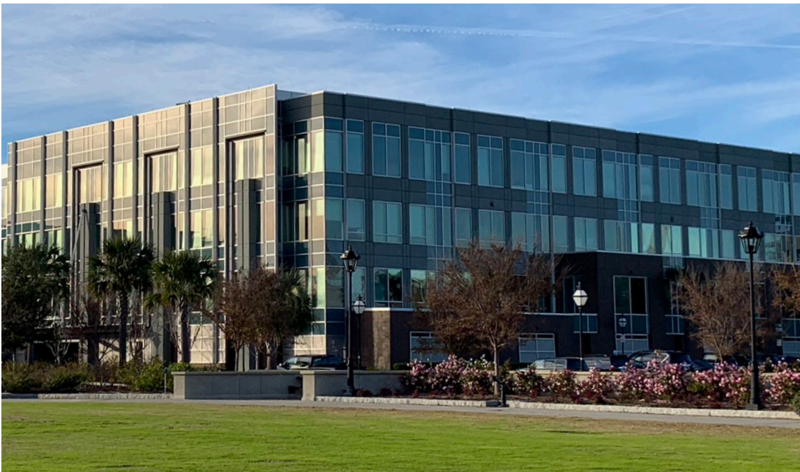
Figure 1. The 25 Calhoun office building at the Calhoun Park Area site (South Carolina).
