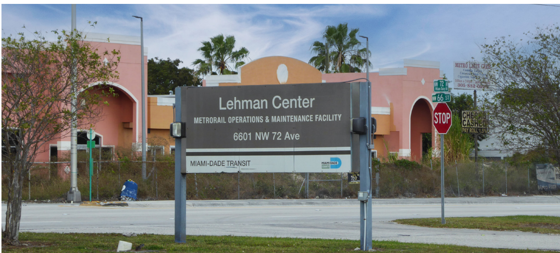
Figure 21. William Lehman Operations and Maintenance Center at the Miami Drum Services site (Florida).
