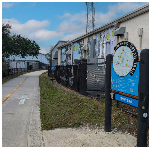
Figures 25 & 26. BarkHaven Dog Bar under construction at the Former Spellman Engineering site (Florida) (left). The Dinky Line segment of the Orlando Urban Trail at the Former Spellman Engineering site (Florida) (right).
