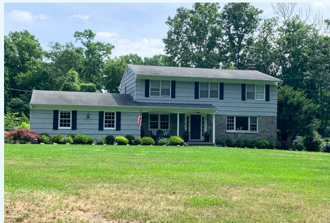
Figure 10. An on-site house at the Smithtown Ground Water Contamination site (New York).
