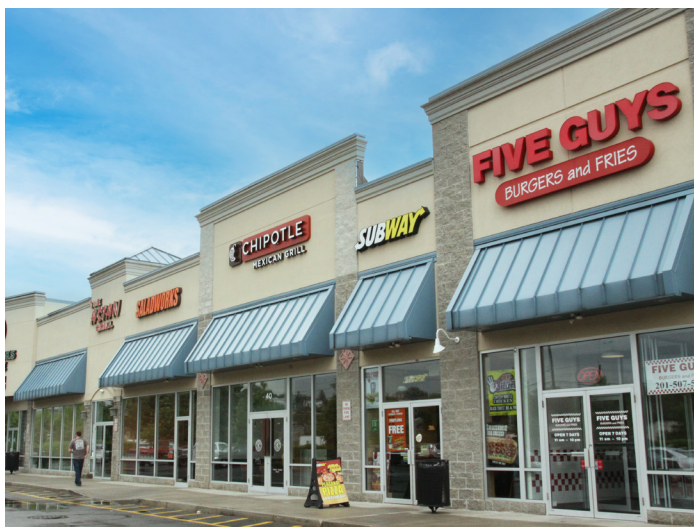
Figure 5: Storefronts at the retail plaza at the Universal Oil Products site (New Jersey).
