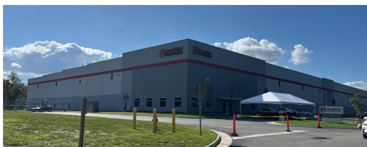
Figure 19. Exterior view of the RoadOne IntermodaLogistics facility at the Former Nansemond Ordnance Depot site (Virginia).
