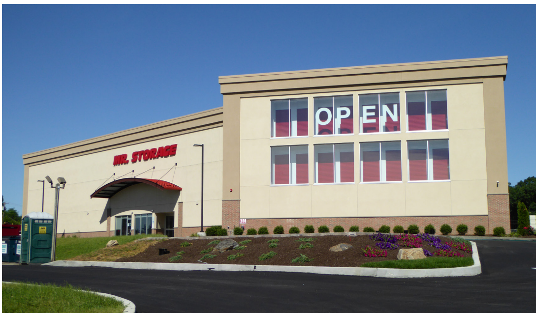
Figure 20. Mr. Storage facility at the Havertown PCP site (Pennsylvania).
