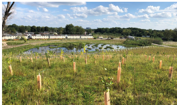
Figure 13. The evapotranspiration cover and mitigation wetland at Eastwick Regional City Park at the Lower Darby Creek Area site (Pennsylvania).
