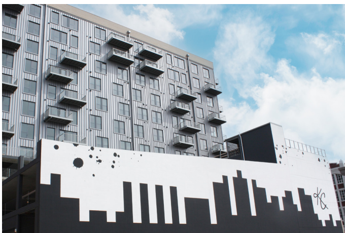
Figure 19. Luxury apartment complex at the PCB Inc. – Missouri site (Missouri, Region 7).
