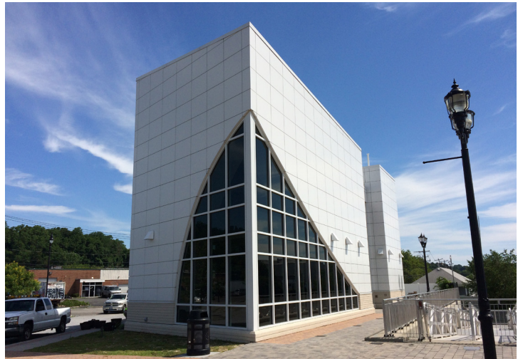
Figure 2. Glen Cove Ferry Terminal at the Li Tungsten Corp. Superfund site. (New York, Region 2).
