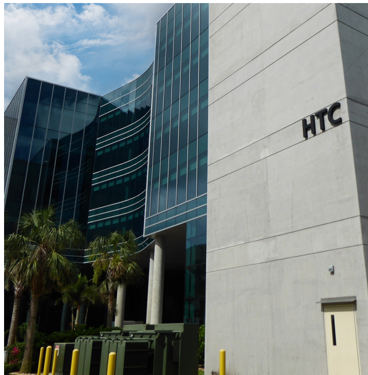
Figure 11. Harris Technology Center at the Harris Corp. (Palm Bay Plant) Superfund site (Florida, Region 4).
