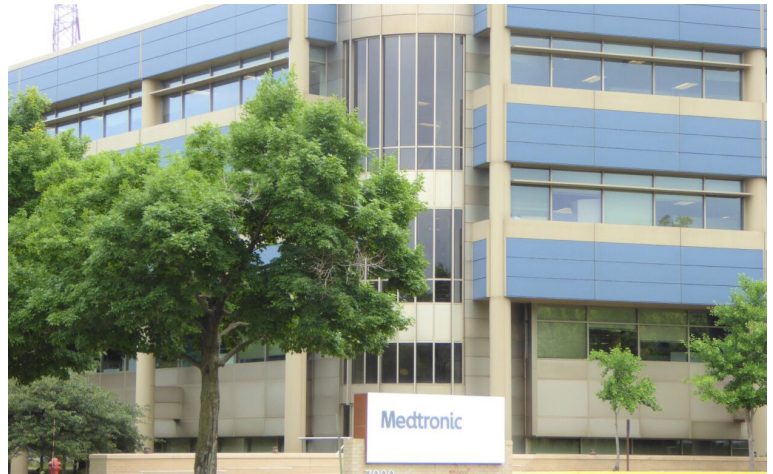
Figure 9. A Medtronic facility at the Boise Cascade/Onan Corp./Medtronics, Inc. site (Minnesota).
