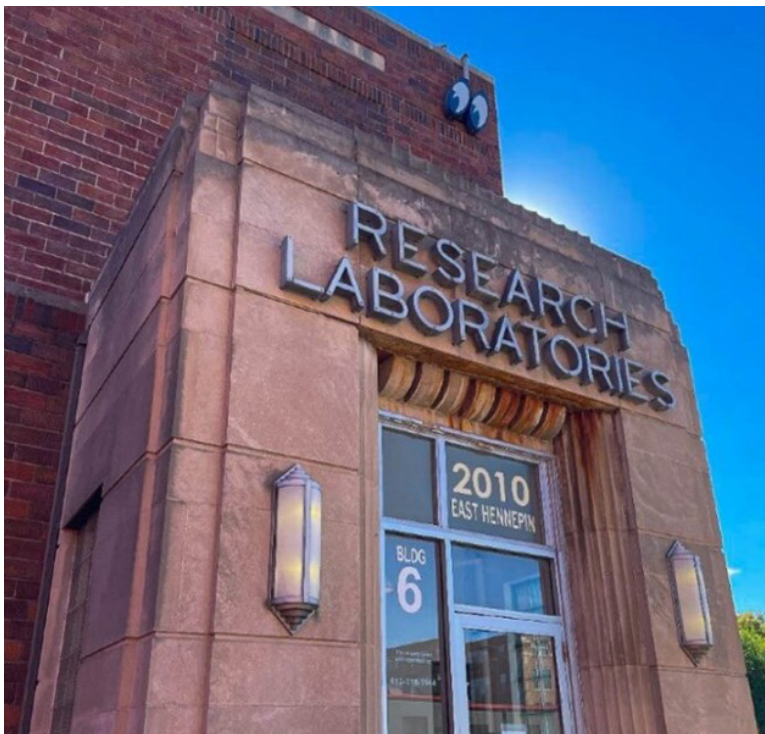
Figure 3. Former General Mills research laboratory facility that now operates as office space on the General Mills/Henkel Corp. site (Minnesota).
