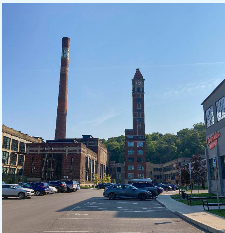
Figure 2. Cartridge Brewing and a former factory building at the Peters Cartridge Factory site (Ohio).
