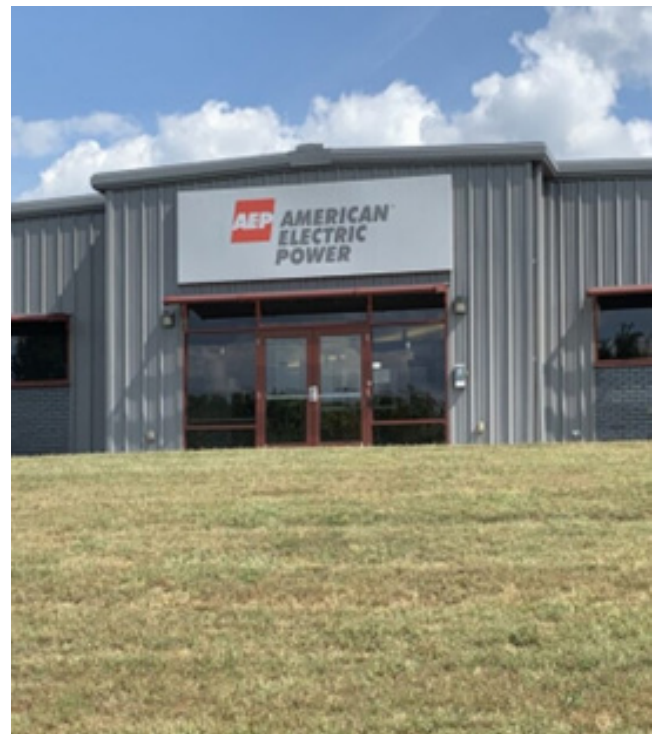
Figure 4. American Electric Power (AEP Ohio) is one of many industrial and commercial businesses operating at the South Point Plant site (Ohio).
