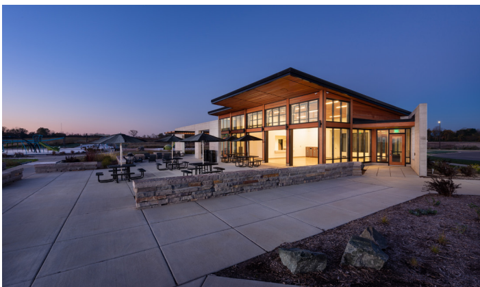
The Larry Haskin Pavilion at Lake Vista Park. (Source: City of Oak Creek)
