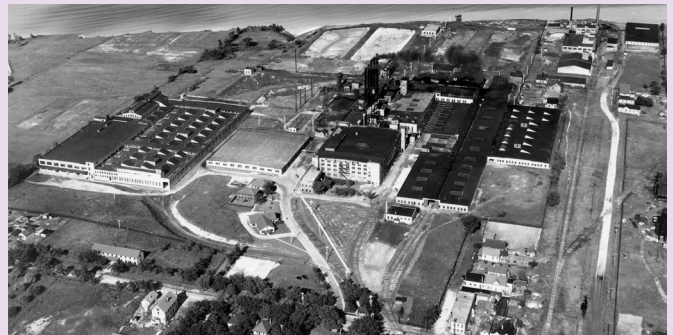
A variety of industries and adjacent neighborhoods made up Carrollville, a hub of factories and plants on the lakefront. (Source: City of Oak Creek)
