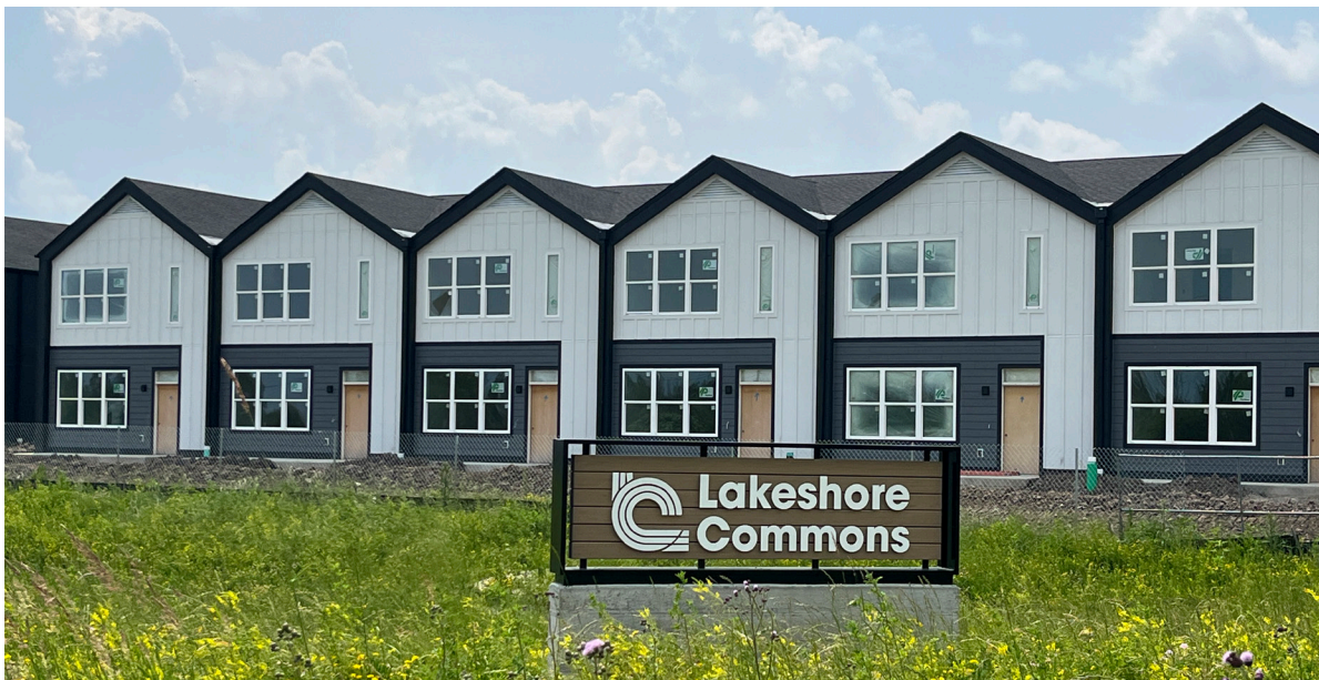
Townhouses under construction in June 2024 at Lakeshore Commons.
