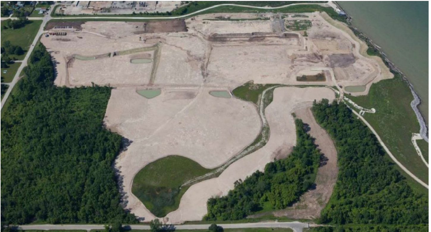
Aerial view of site cleanup, 2013. (Source: EPA)
