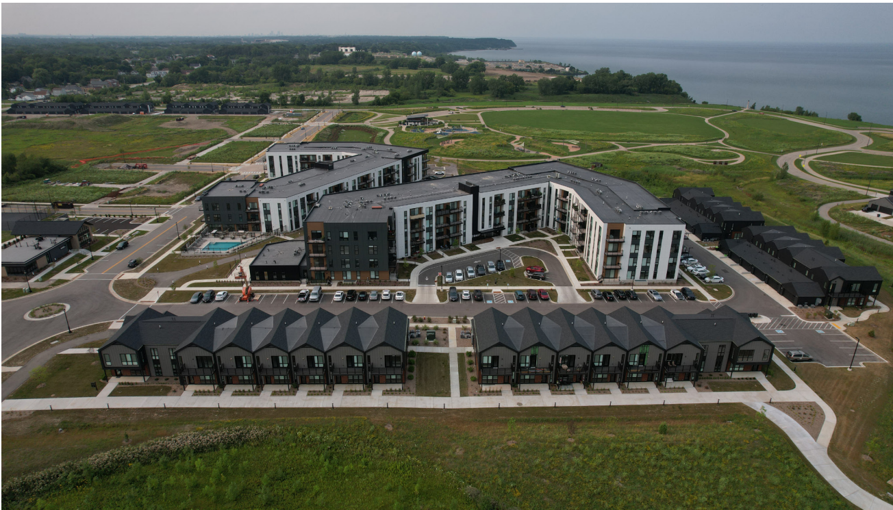
Aerial view of Lakeshore Commons under construction in August 2024. (Source: F Street)
