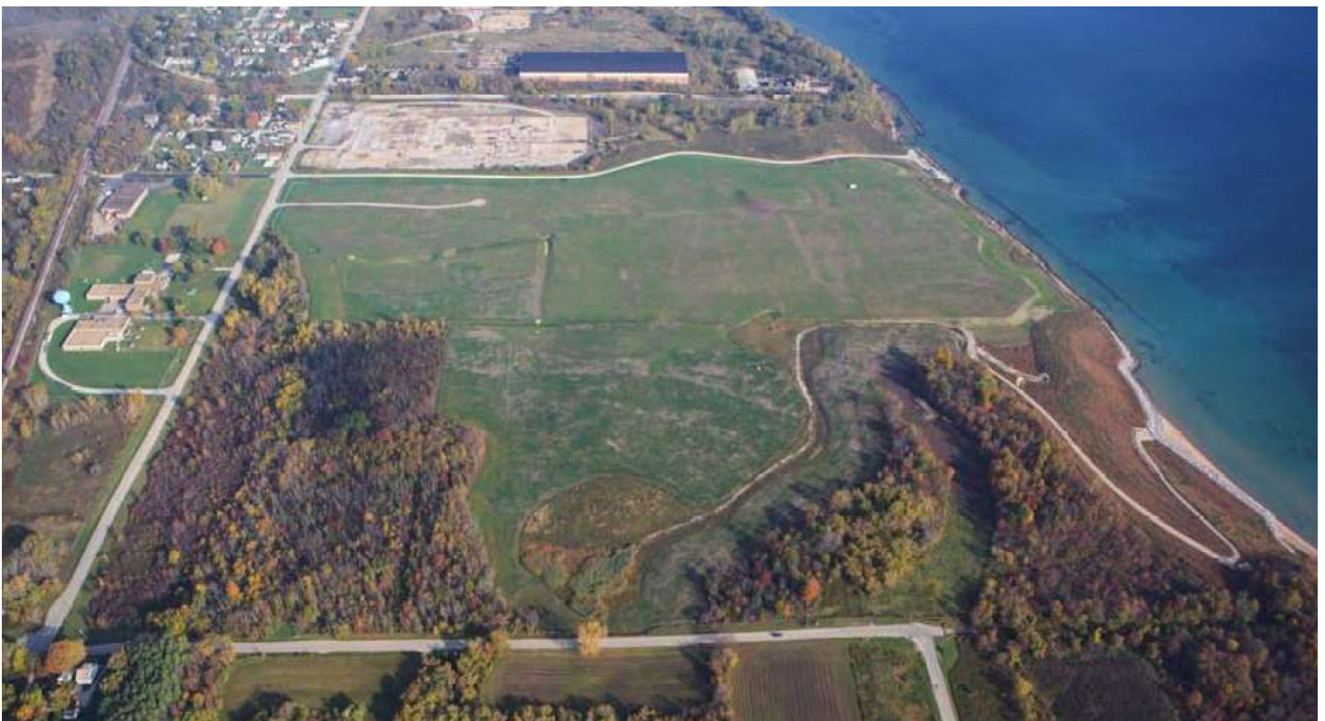
Aerial image of vegetative regrowth at the site. (Source: EPA)
