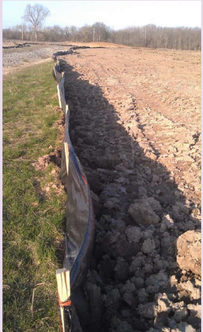
Ground-level view of some of the clean soil trucked in from Milwaukee that served as capping material and the foundation for Lake Vista Park. (Source: EPA, 2013)
