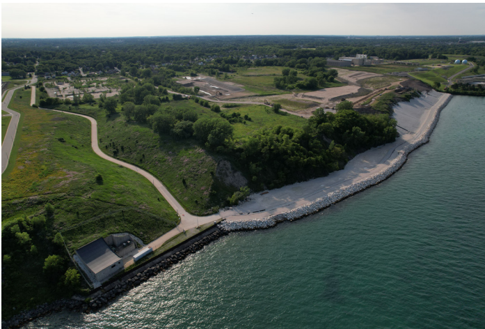
Aerial view of the North Bluff Stabilization Project. (Source: F Street)
