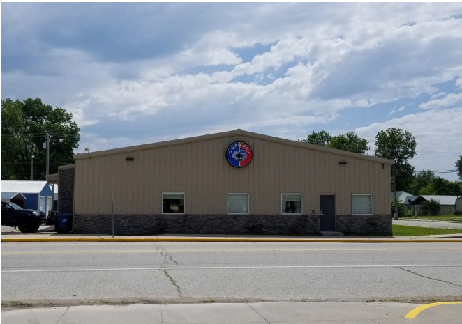
Figure 4: Environmental Realty Building.
