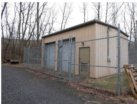
The groundwater extraction and treatment building at the Drake Site.
