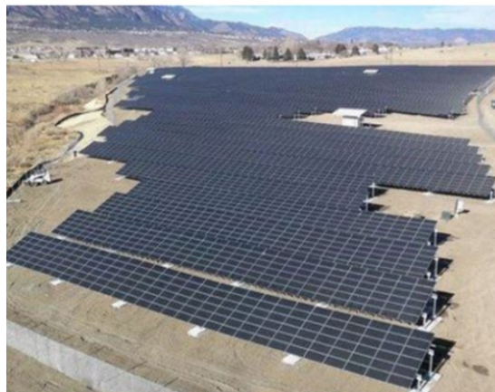
Fig. 7 Ballasted solar system. Source: NREL.
