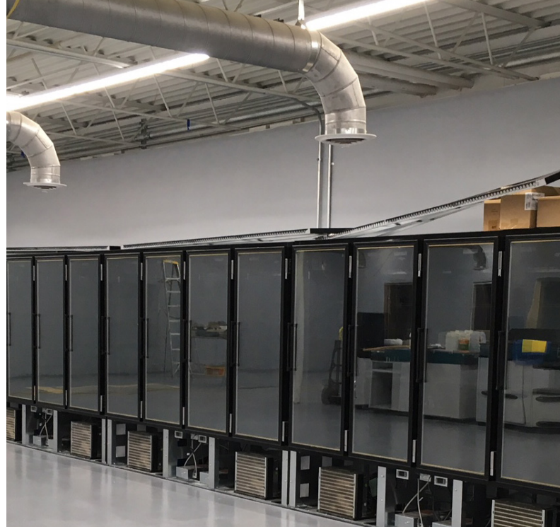
New equipment installation at city-owned grocery store located in Downtown Caney.
