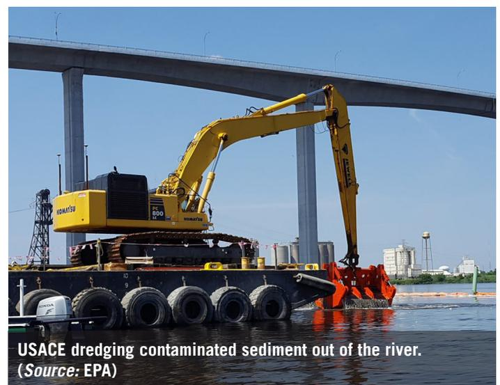
USACE dredging contaminated sediment out of the river. (Source: EPA)
