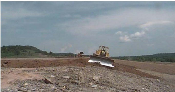
Cover soil placement. (Source: ODEQ)
