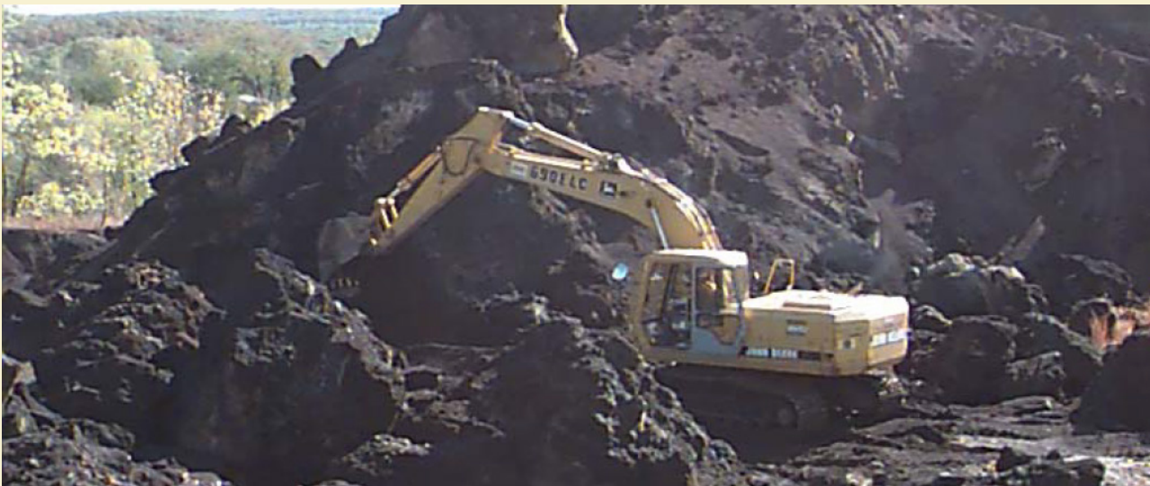
Slag pile cleanup on site. (Source: ODEQ)
