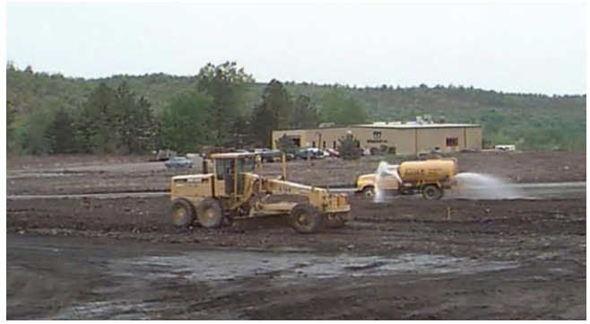
Final site grading. (Source: ODEQ)
