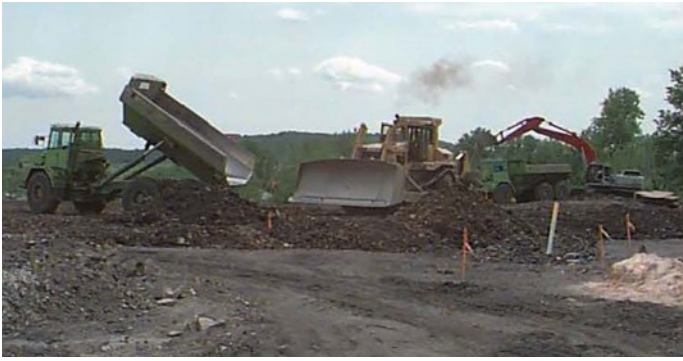
Filling in excavated areas with clean material. (Source: ODEQ)
