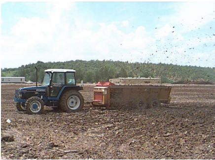
Cover soil placement. (Source: ODEQ)
