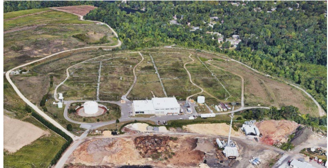
Figure 8. Aerial view of the OU1 containment system and the OU2 groundwater and leachate treatment facility. (Source: 2019 Google Imagery, 2019 Maxar Technologies, U.S. Geological Survey, USDA Farm Service Agency, map data 2019)
