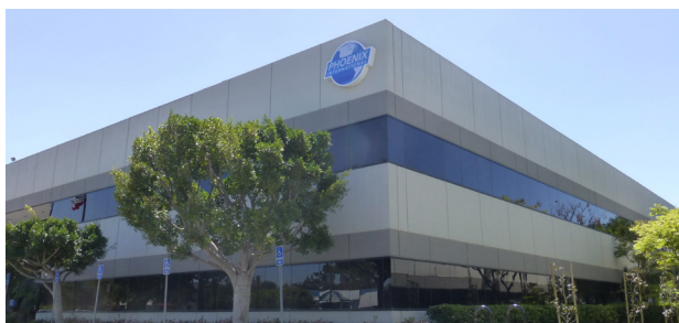
Figure 84. Commercial reuse at the Del Amo site (California, Region 9).
