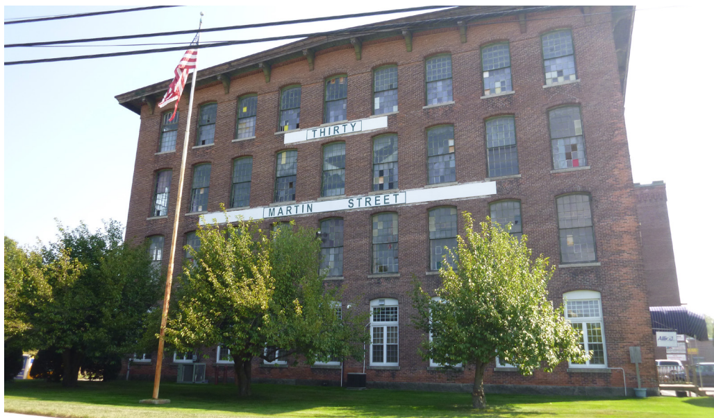
Figure 10. The 30 Martin Street building is home to several small businesses at the Peterson/Puritan, Inc. site (Rhode Island).
