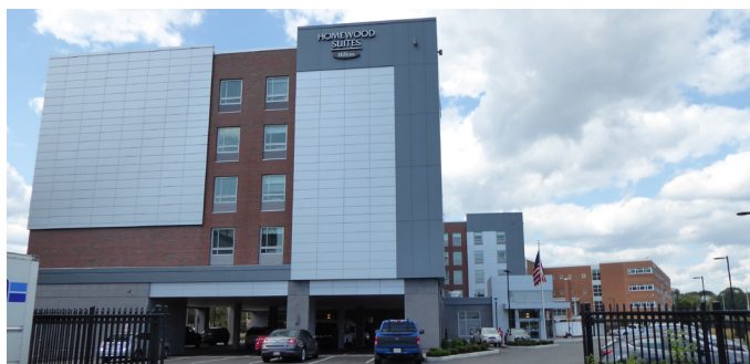
Figure 32. Homewood Suites at the Lawrence Metals (Former) site (Massachusetts, Region 1).
