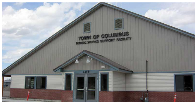
Figure 79. The town of Columbus' public works building at the Mouat Industries site.
