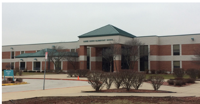
Figure 61. Public service uses, including this elementary school, are located at the U.S. Smelter and Lead Refinery, Inc. site.
