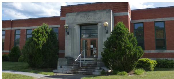
Figure 44. The former American Viscose Corporation administrative building at the Avtex Fibers site has been refurbished and now supports several small businesses (Virginia, Region 3).
