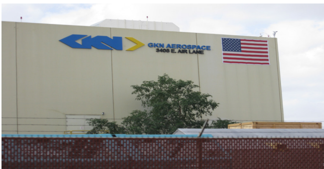
Figure 85. Active aerospace manufacturing facility at one of the source areas at the Motorola, Inc. (52nd Street Plant) site.
