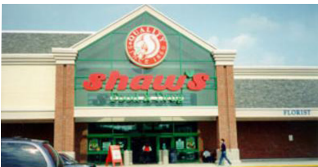
Figure 34. Reuses at the Bangor Gas Works site include a Shaw's Supermarket and Pharmacy.
