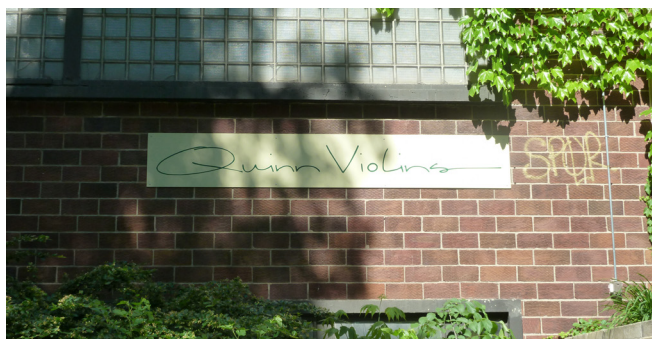
Figure 63. Business located at the General Mills/Henkel Corp. site.
