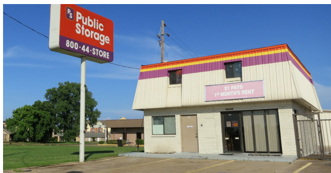
Figure 68. Many businesses continue to operate at the Highway 71/72 Refinery site, including this storage facility.
