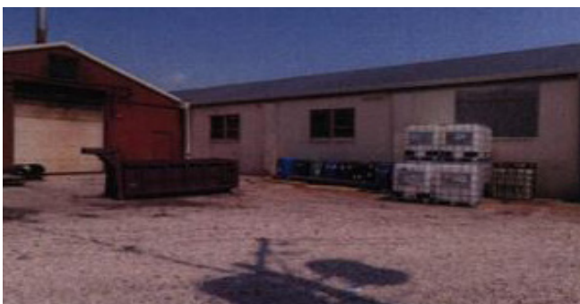
Figure 73. This metal-plating facility continues to operate at the Electro-Coatings, Inc. site.
