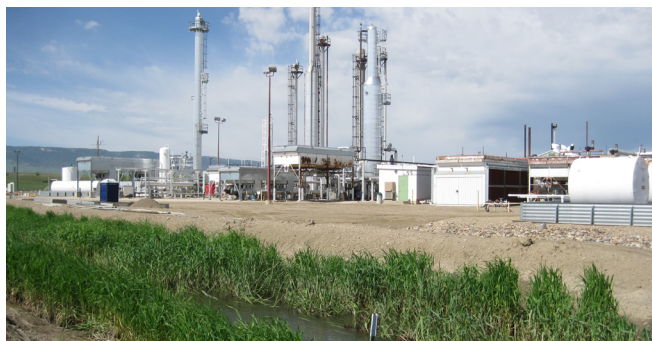
Figure 83. An active gas compression facility at the Mystery Bridge Road/U.S. Highway 20 site.
