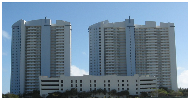
Figure 52. The two residential towers at the Munisport Landfill site.
