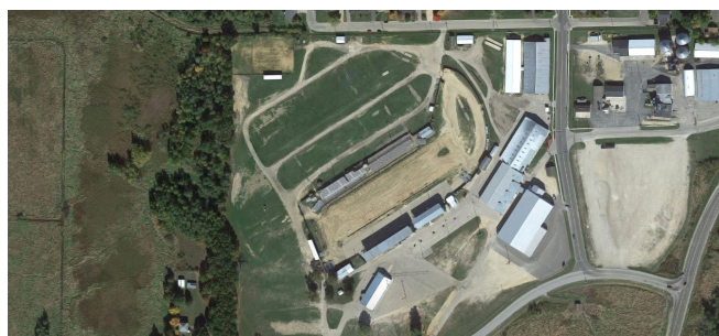
Figure 65. Aerial view of the Tomah Fairgrounds site. Imagery © 2019 Google.
