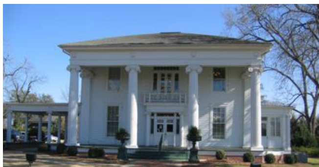
Figure 53. Entrance to the welcome center at the Woolfolk Chemical Works, Inc. site.
