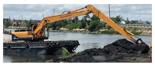
In 2019, EPA completed its 15th and final season of dredging, hydraulic transport, and shipment of dewatered, highly contaminated PCB subtidal sediment from New Bedford's Upper Harbor. EPA:
