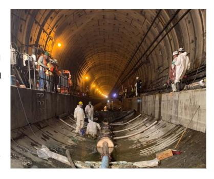
monitoring locations, and sulfuric acid was detected at the two monitoring stations located at the tunnel's entrance. Over 110,000 gallons of liquid were pumped from the sump area and sent for disposal over a series of days.
