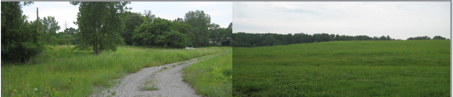
Images from left to right: An access road on the property and a view of the landfill cap.
