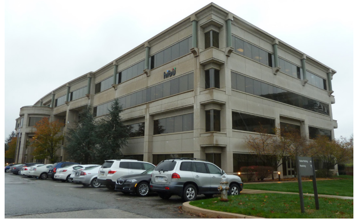
Figure 6. Commercial reuse at the Crater Resources, Inc./Keystone Coke Co./Alan Wood Steel Co. site (Pennsylvania).
