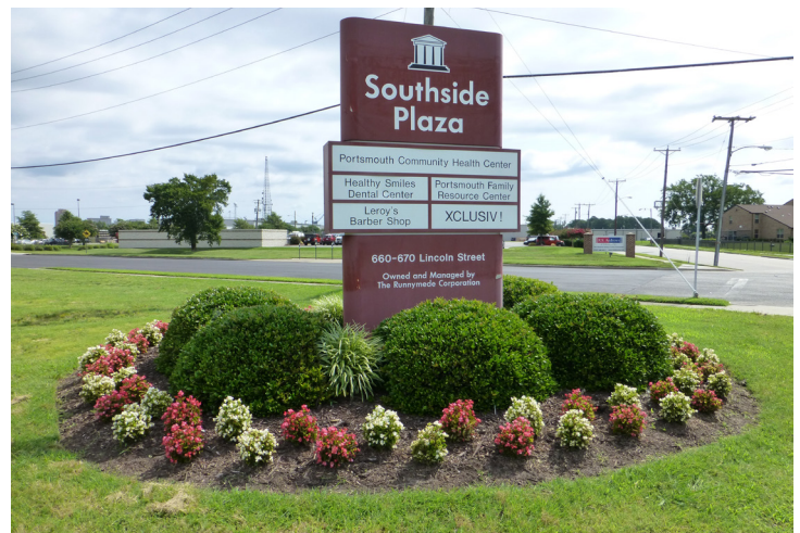
Figure 2. Entrance to the Southside Plaza business park at the Abex Corporation site (Virginia).
