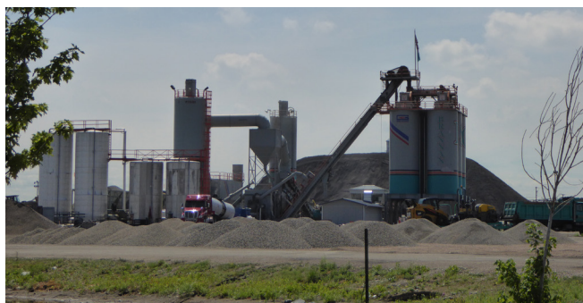
Figure 18. Brannan Sand & Gravel's asphalt plant at the Broderick Wood Products site.
