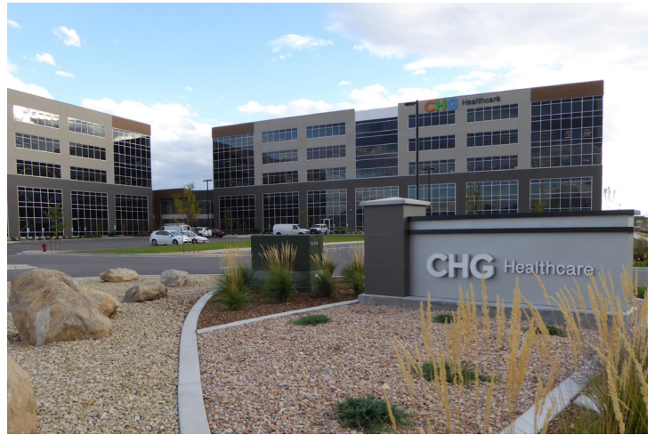
Figure 2. The new CHG Healthcare Services corporate headquarters facility at the Midvale Slag site (Utah).
