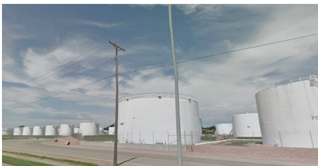
Figure 21. Petroleum storage tanks at the Williams Pipe Line Co. Disposal Pit site.
