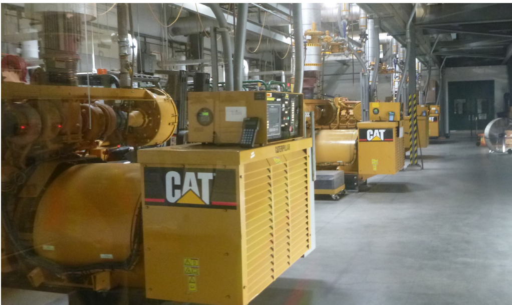
Figure 13. The landfill gas-to-energy plant at the Lowry Landfill site converts landfill gases to electricity (Colorado).
