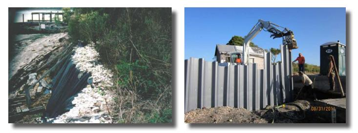
A total of 220 linear feet of sheet pile at the site prevents erosion, protecting the shell midden and other cultural and environmental resources.
