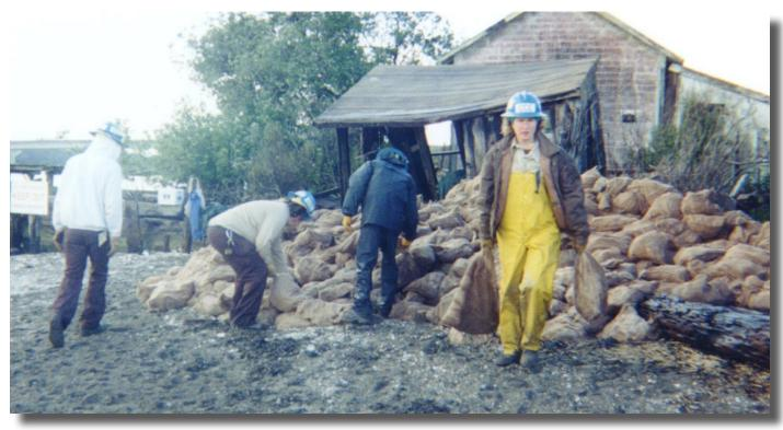
Workers using oyster shells for erosion control.
