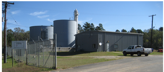
The site’s groundwater treatment plant will continue to operate for the foreseeable future.
