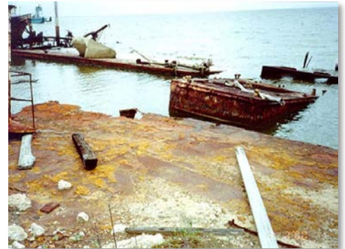
Figure 3. Historical photo showing the State Marine site before cleanup.
