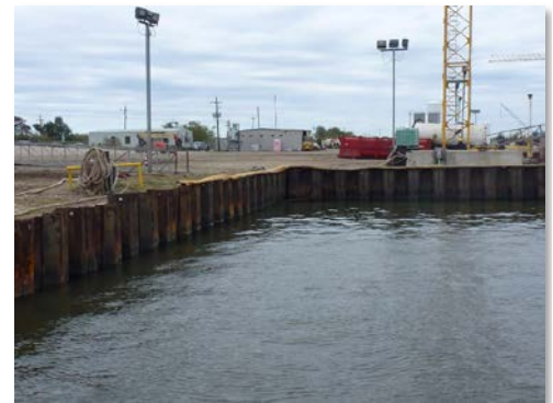
Figure 9. View of the barge docking area for Tubal-Cain Gas Free Services.
