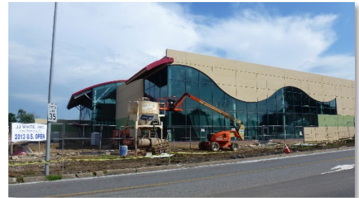
Figure 6. Construction of the YMCA facility.
