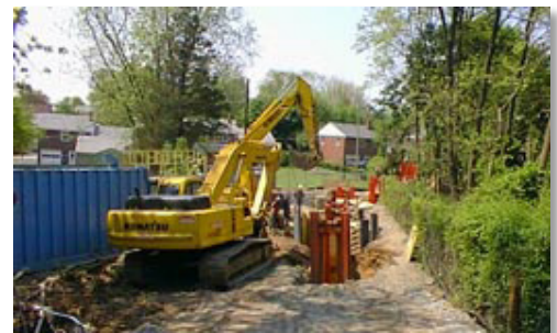
Figure 4. Cleanup activities at the Havertown PCP site.
