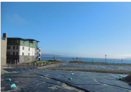
Figure 16: Construction of capped surfaces at the Asarco Inc. site (Washington)
