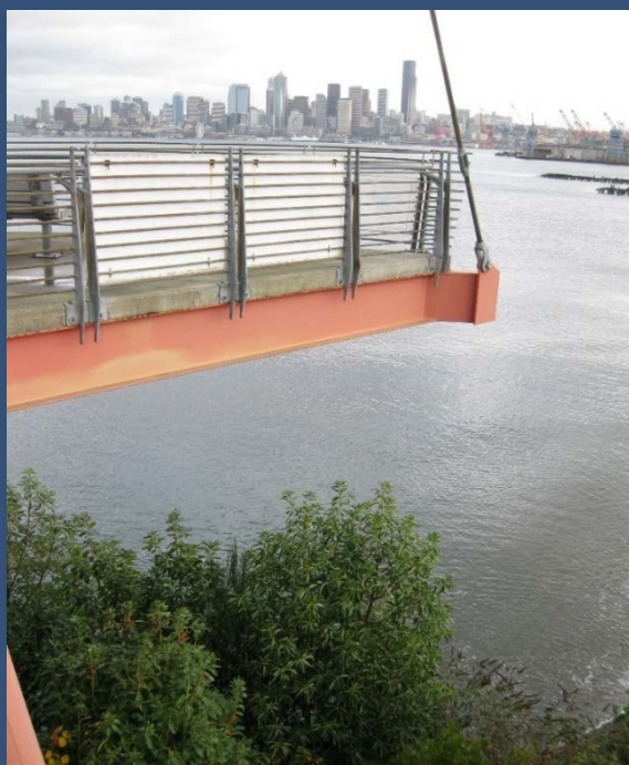
Figure 2: View of the Seattle skyline from Jack Block Park, located on the Pacific Sound Resources site (Washington)
