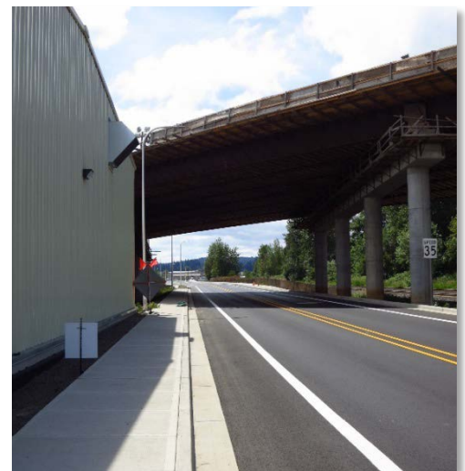
Figure 12: Sunrise Corridor connector extending over new street, next to the ODOT maintenance facility at the Northwest Pipe & Casing/Hall Process Company site (Oregon)
