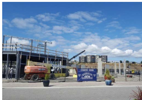
Figure 17: Construction underway at the Asarco Inc. site (Washington)
