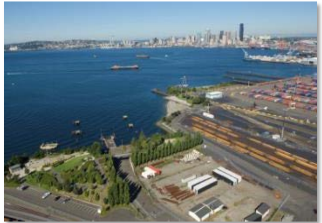
Figure 13: Part of the container terminal facility and public shoreline access area at the Pacific Sound Resources site (Washington)
