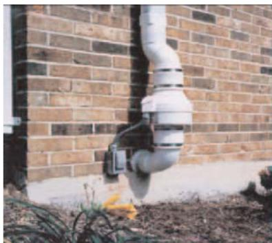
**Sub-slab mitigation system:** This system draws radon and other vapors out of the soil and vents them outside
