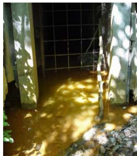
Acid mine drainage leaking from the Stowell portal at Mammoth Mine, California.
