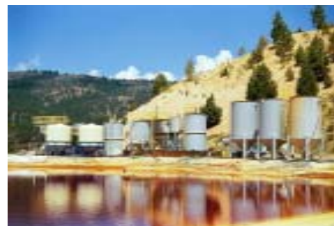
Bi-phasic chemical treatment system of acid mine drainage at Leviathan Mine, California.
