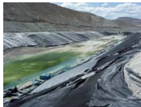
Inactive copper leachate collection pond adjacent to heap leach pile (left) at the Anaconda Mine, Yerington, Nevada.
