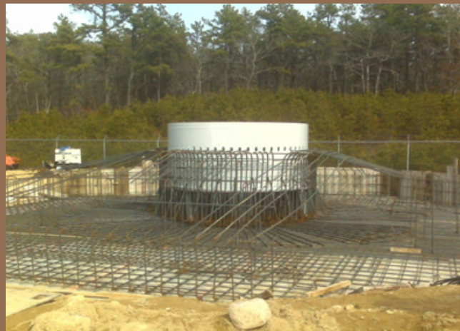
Construction of wind turbine foundation at Massachusetts Military Reservation (March 2009) (source: Massachusetts Military Reservation Cleanup Team)
