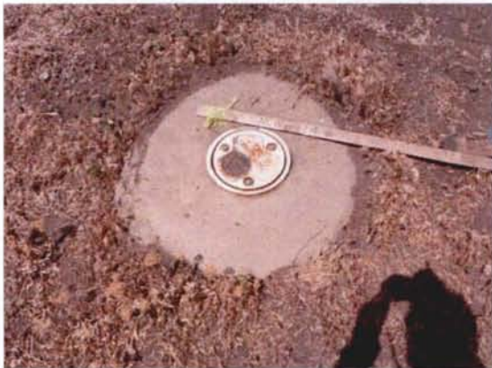
Monitoring well W-14
