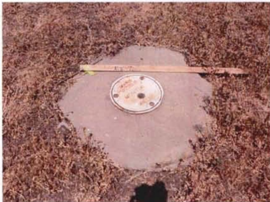
Monitoring well W-7
