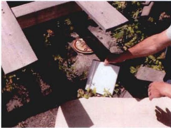
Monitoring well W-13
